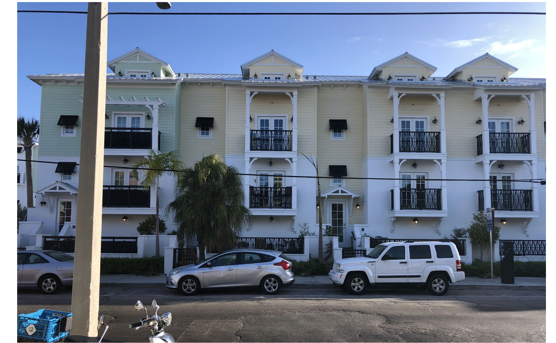
SAMPLE ELEVATION TAKEN AT 127-135 SIMONTON STREET (SAMPLE ONLY, INDICATIVE OF SIMILAR DETAILING, MATERIALS, AND COLORS)
