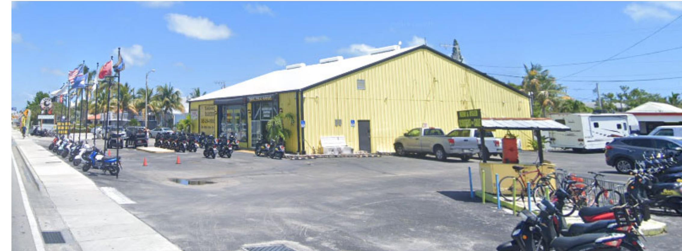
1910 N. ROOSEVELT BLVD. (TO BE DEMOLISHED)
