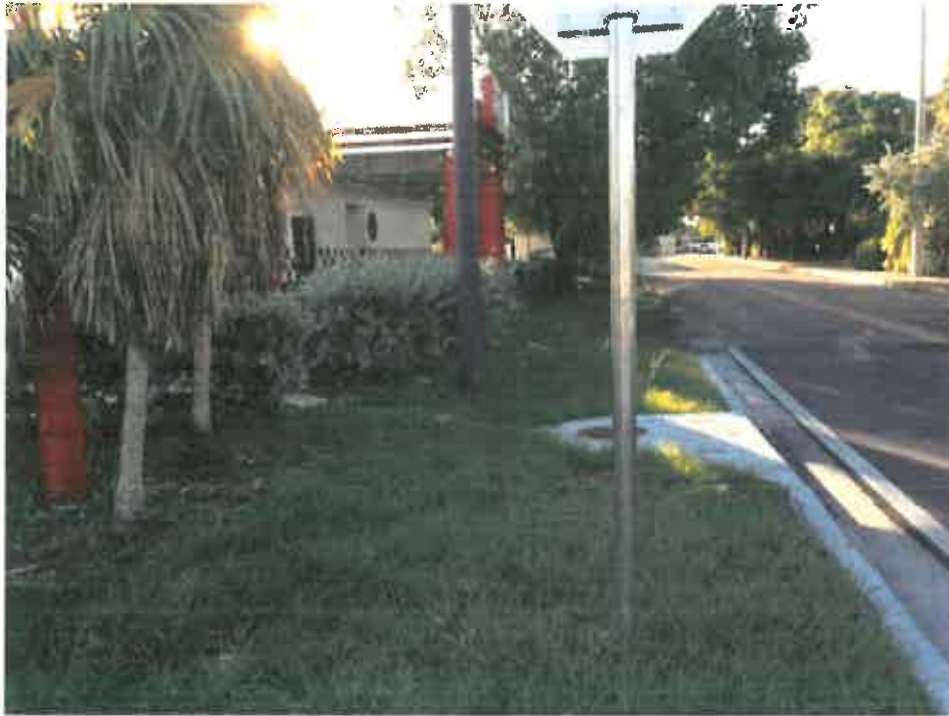
Existing Strip between Curb Mature Buttonwood Hedge and 7 th Street to be utilized for the drainage swale.
