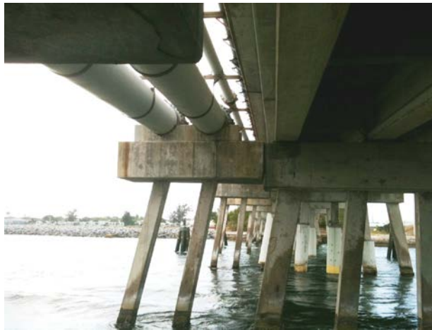
The City of Key West Sewer Bridge is the two pilings and concrete support for the two pipes on the left of the picture. It sits immediately adjacent to the Navy's roadway bridge to Fleming Key
