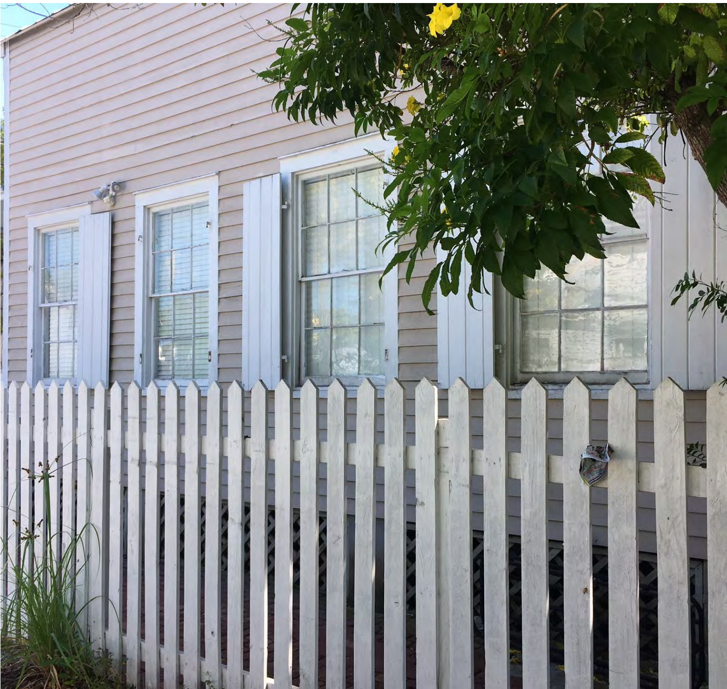
Four of the windows proposed to be replaced.
