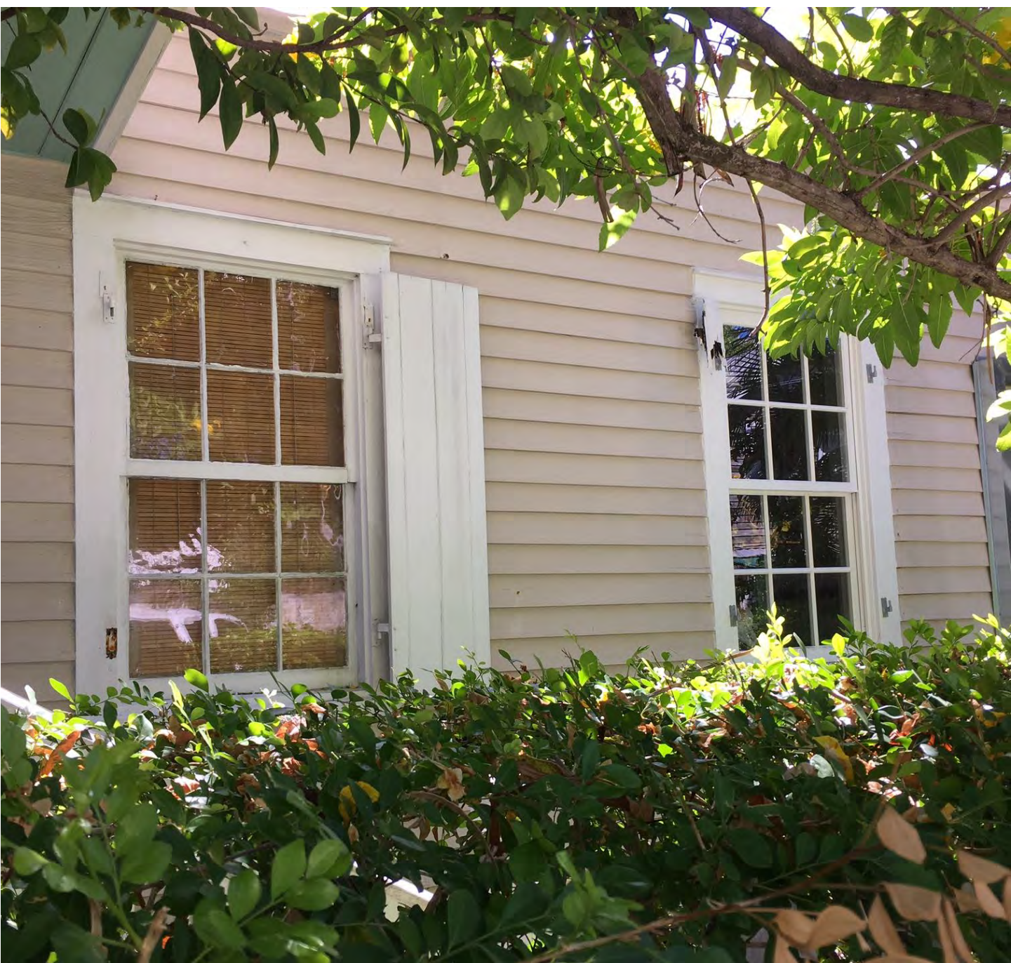
Window #5 with a new Lincoln 6/6 window
