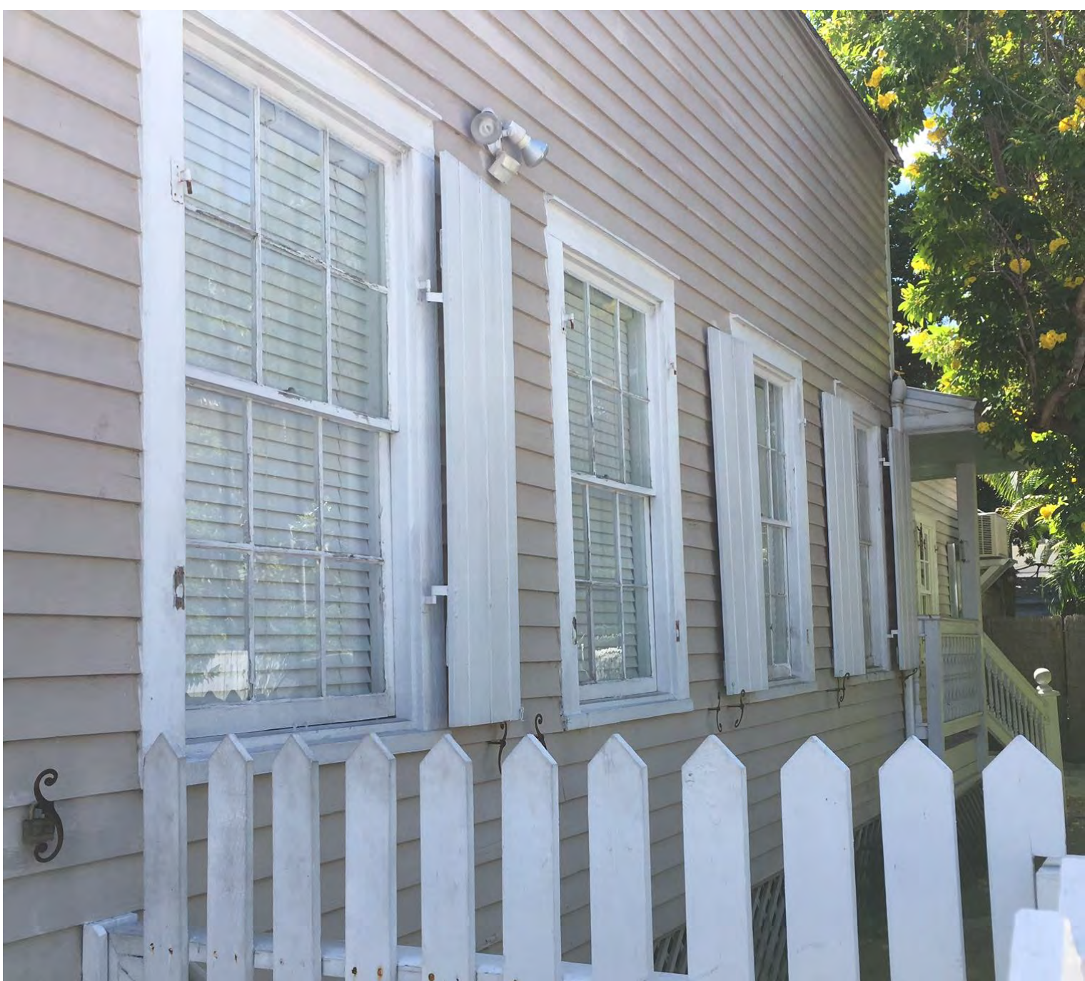
Four of the windows proposed to be replaced.
