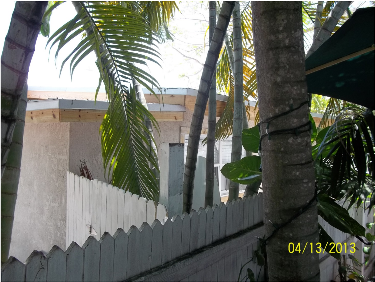
Unpermitted fence added to block entry from front tenant
