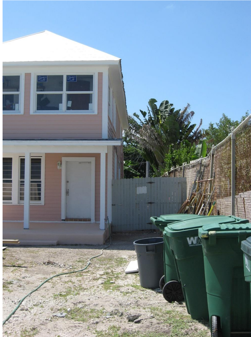
404 South Street before changing to 5 V-Crimp roofing.
