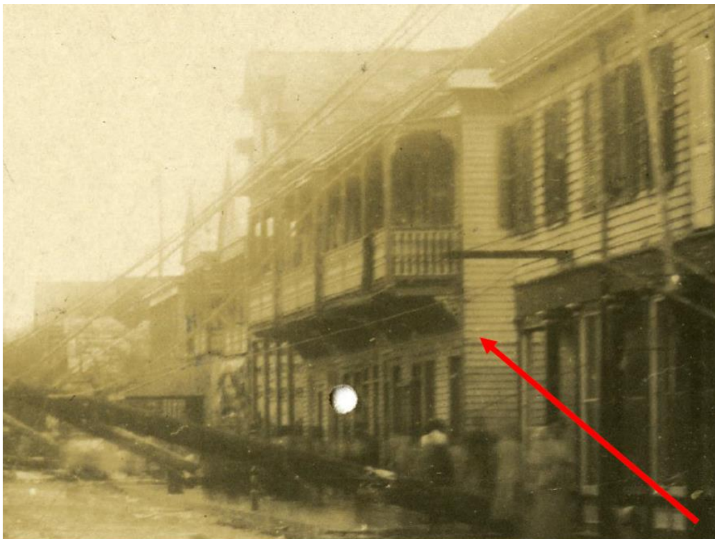
Historic photo from 1909 showing 210-216 Duval Street with wood lap siding and three second-story porches facing Duval Street.
