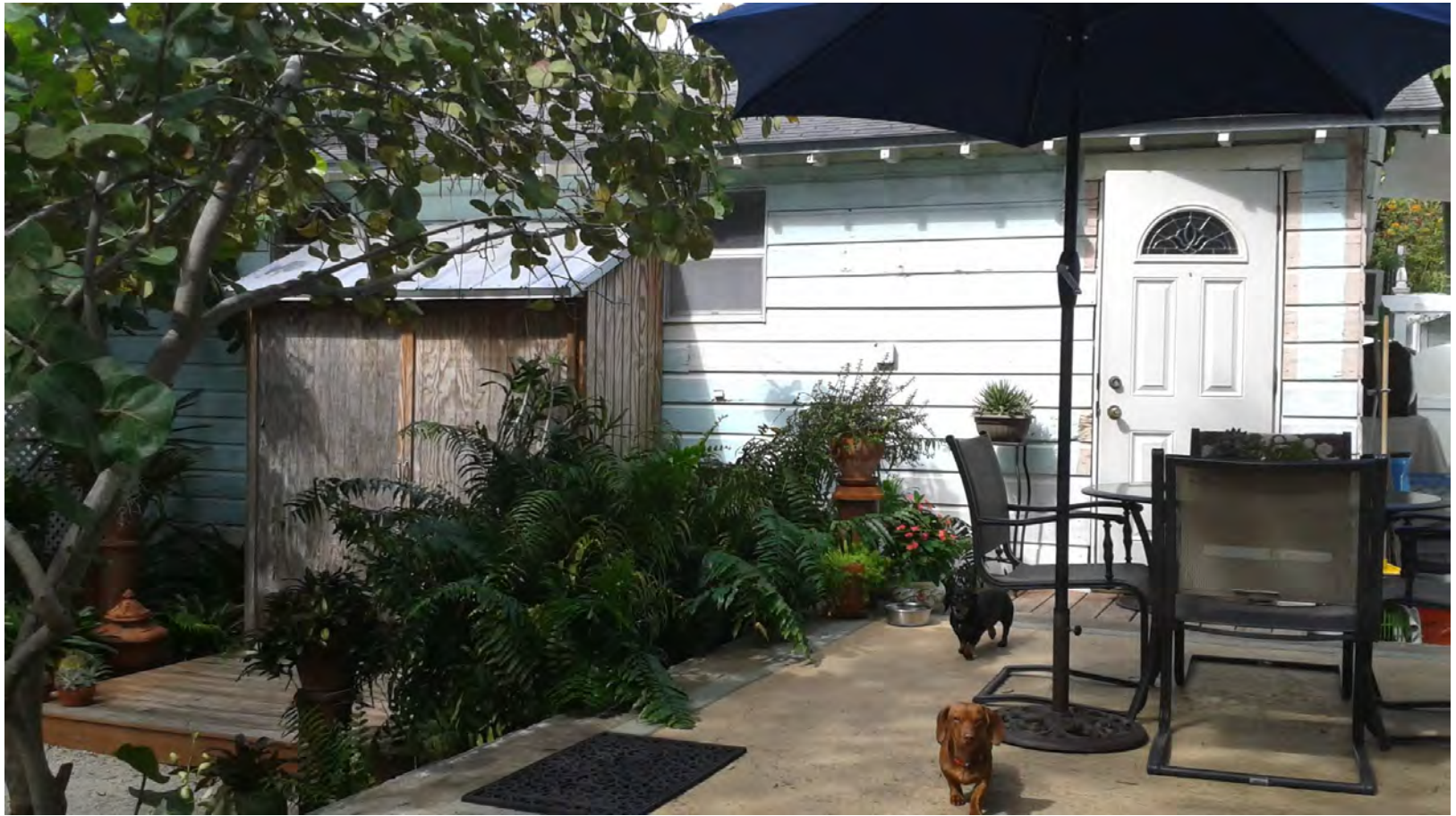
512 Amelia (extant), rear with utility lean-on, and cement-block and slab deck.
