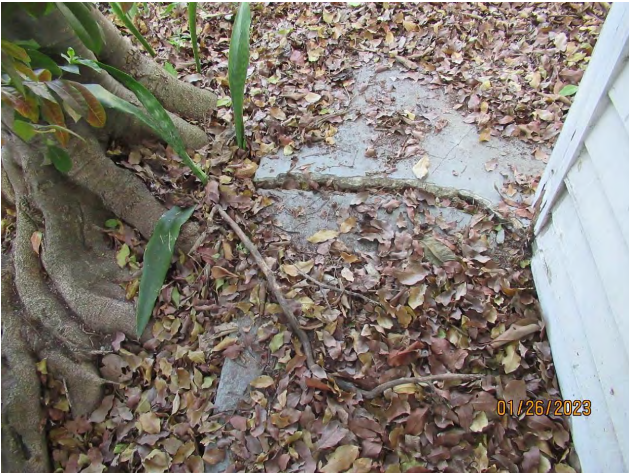
Photo of base of tree closest to existing structure.
