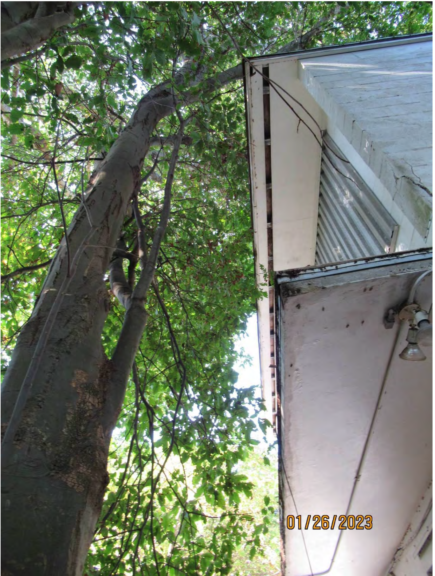
Photo of tree trunk and existing structure (structure to be demolished).
