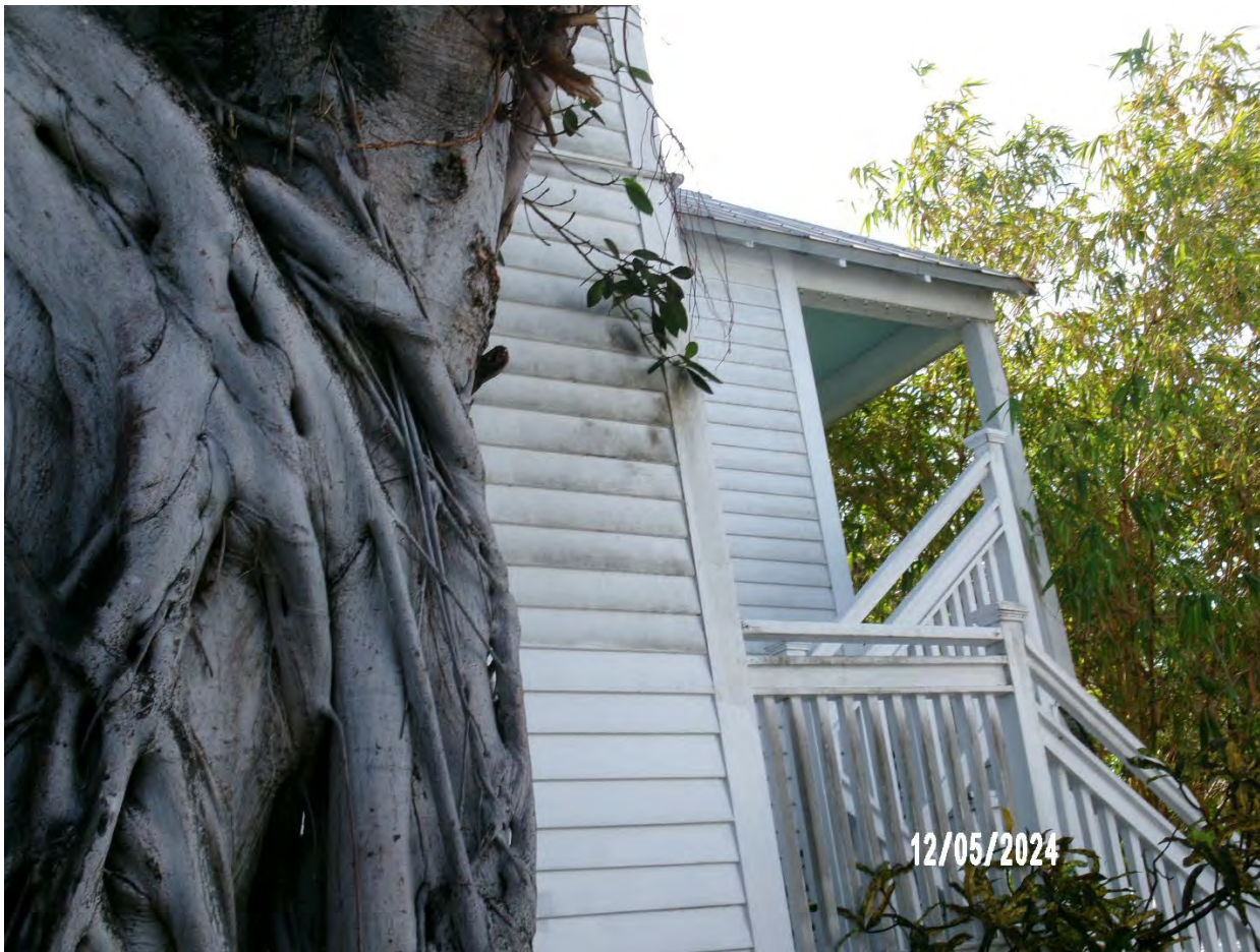
Photo showing discoloration of siding on structure from tree- possible sooty mold (by product of white fly).
