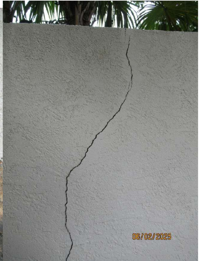
Second crack on west wall of property. Also appears to have been previously patched and painted.
