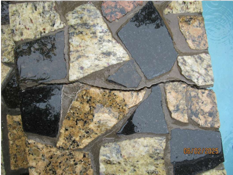
Crack leading up to pool retaining wall and on coping.
