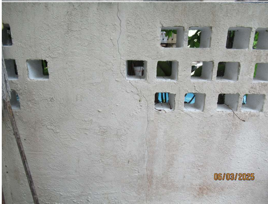
Crack in wall on West side of property. Looks like it had been previously patched and painted.
