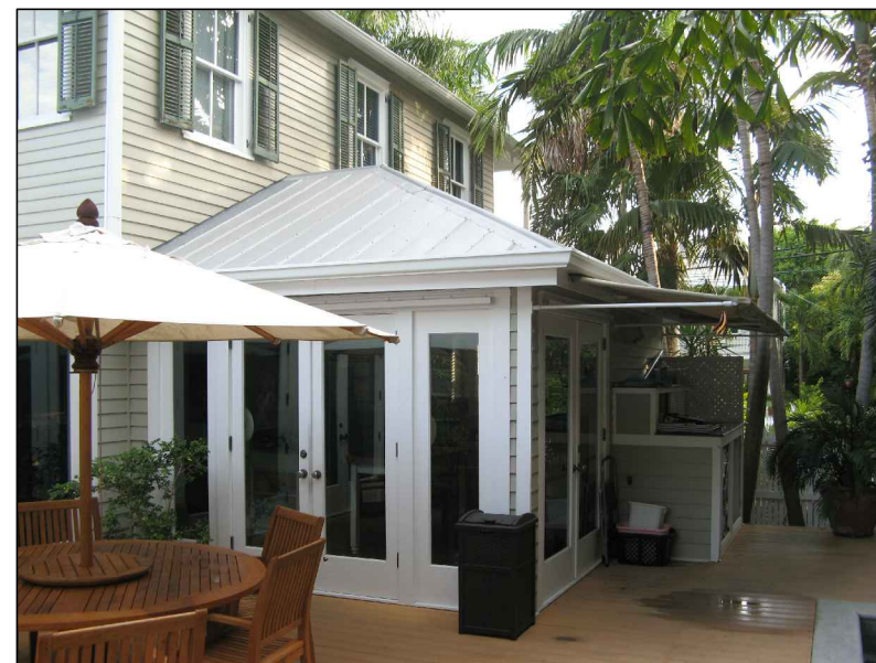
EXISTING KITCHEN ADDITION
