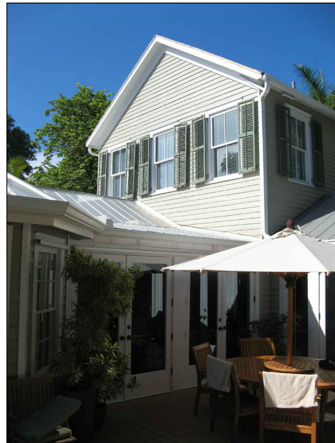
VIEW OF EXISTING HOUSE FROM COURTYARD
