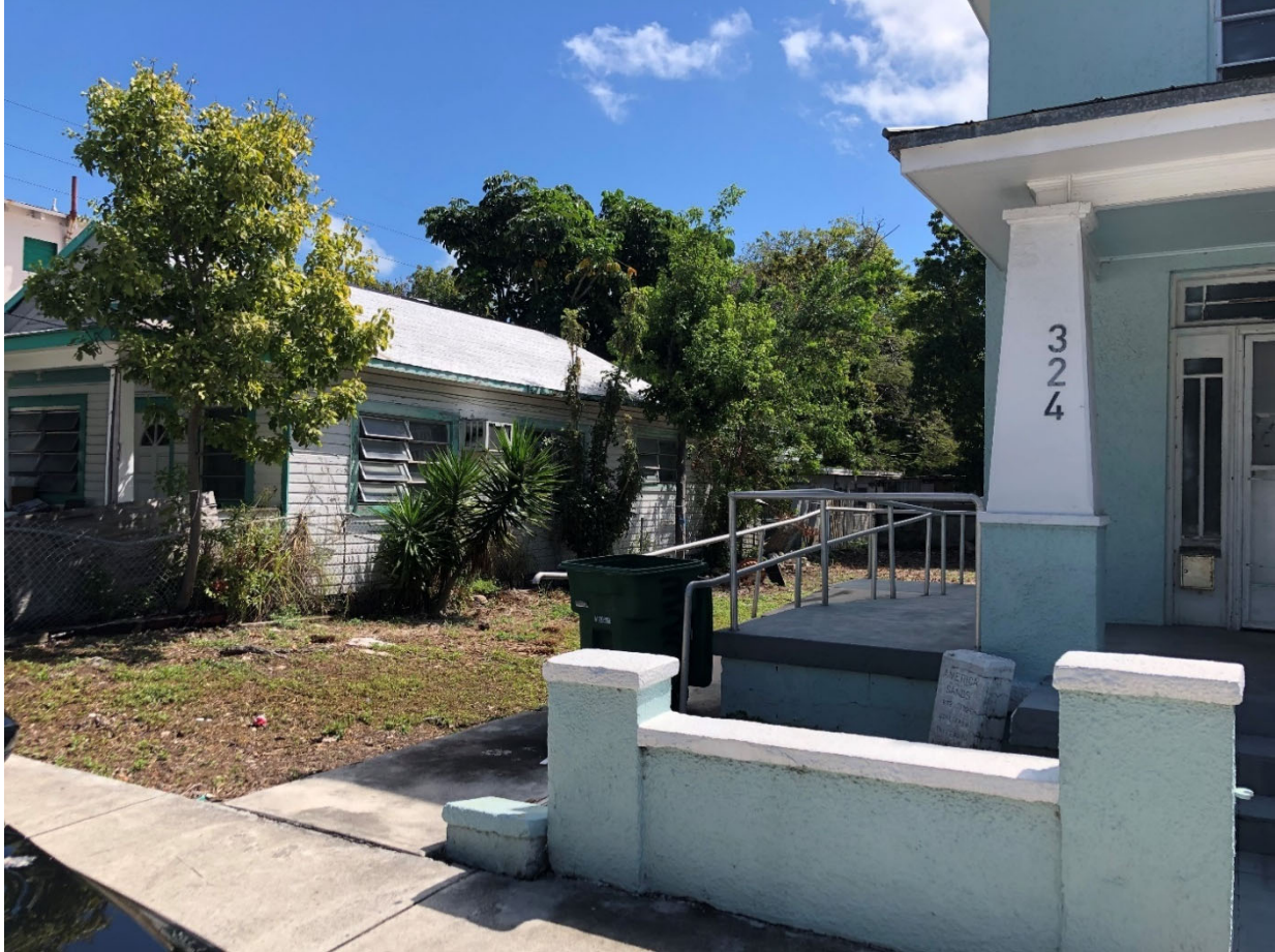
Street View of 324 Truman and 326 Truman, to the left, from Truman Ave
