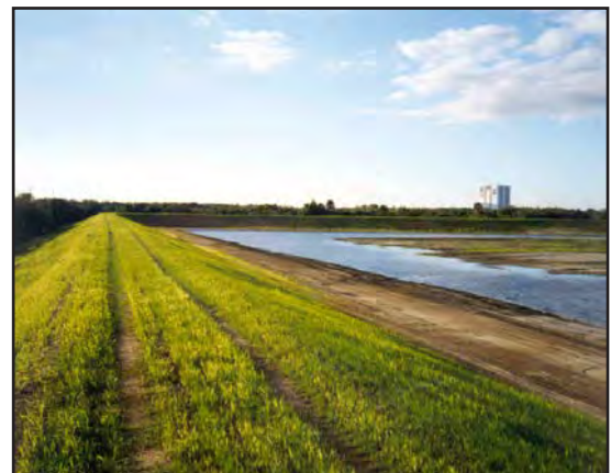
Levee at Placement Site2B
