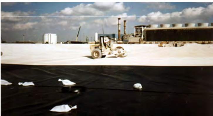
Geosyntec provided CQA services for an ash monofill liner system.
