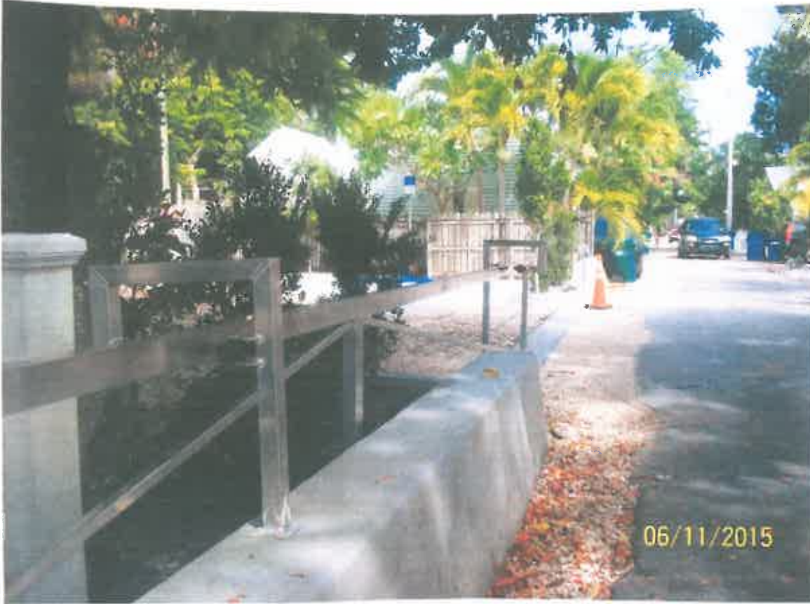
Concrete wall that is the subject of this easement application.
