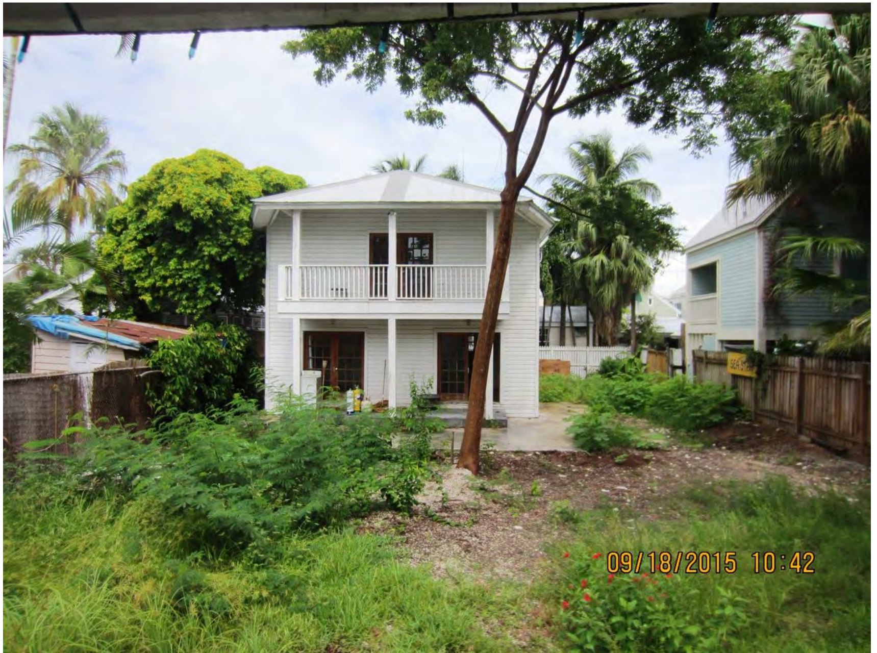
Front of existing guesthouse.
