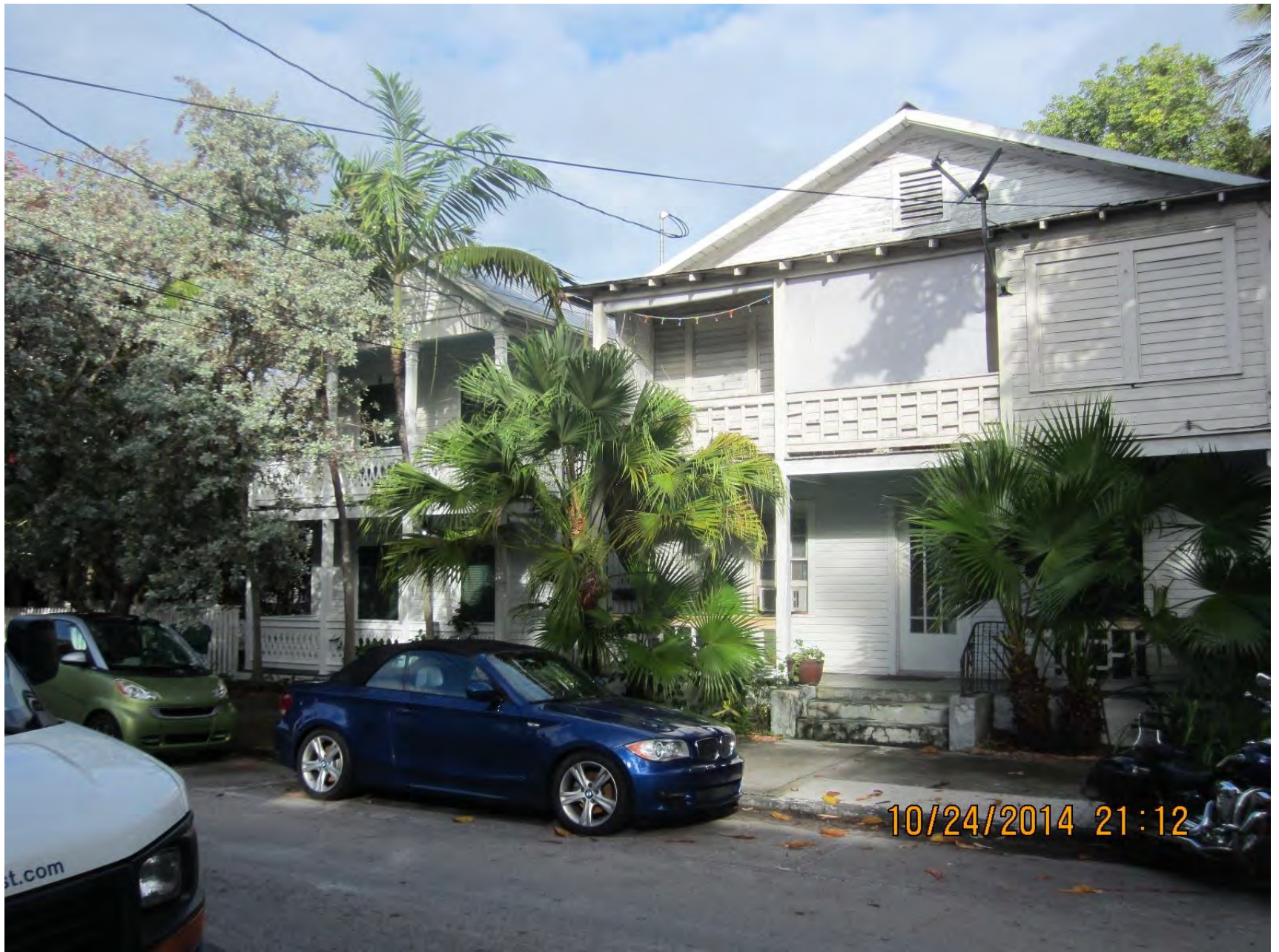
Neighboring Structures on Fleming
