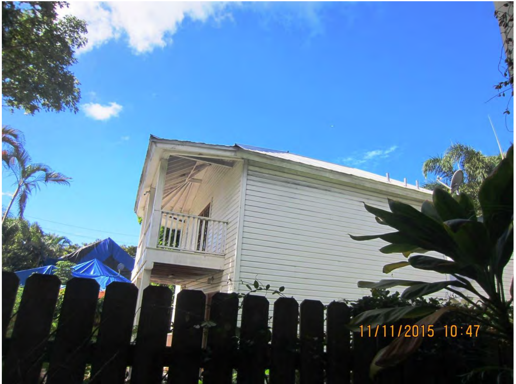
Side of existing guesthouse from Stickney Lane.
