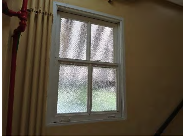
Photo 20: Metal framed fire rated windows in the stair shafts.
