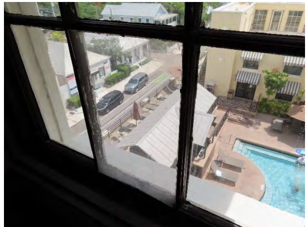
Photo 6: Missing glass pane was replaced with plexiglass.
