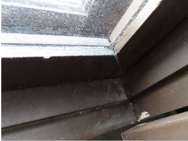
Photo 8: Interior glazing panes appeared to be tempered glass.
