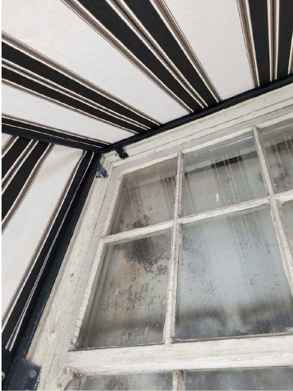
PHOTO 6: Installation of awning attached to window frame
