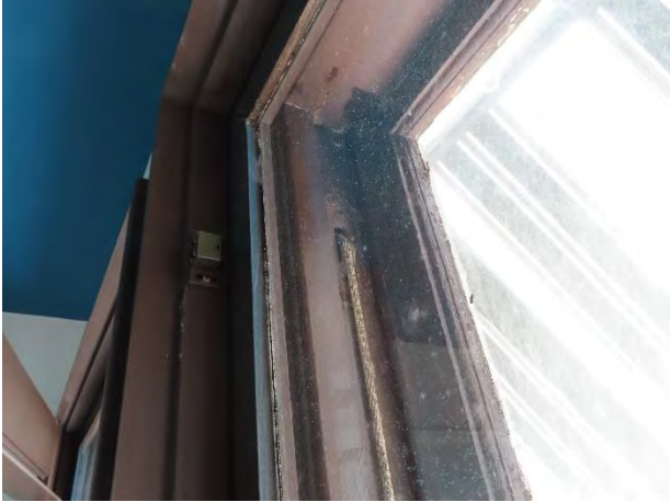
Photo 7: Interior secondary glass glazing, typical in rooms along Duval Street.
