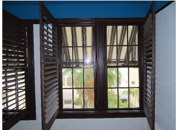
Photo 4: Typical window assembly.
