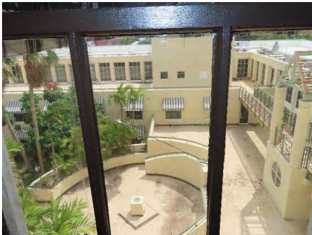
Photo 5: Fractured pane in room 548.
