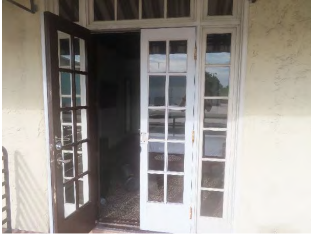
Photo 1: Overall view of the balcony doors on the second floor.
