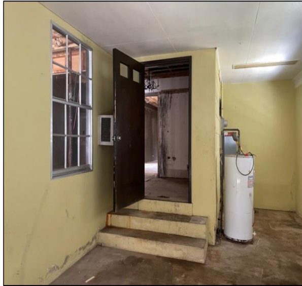
Interior of garage 2021
