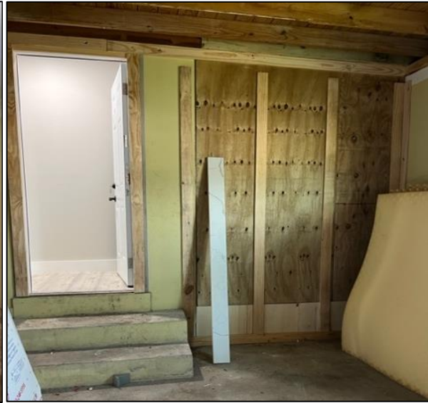
Interior of garage 2023
