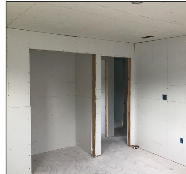
Addition of walls to create closets
