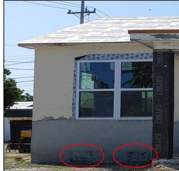
Covering of flood vents 2021
