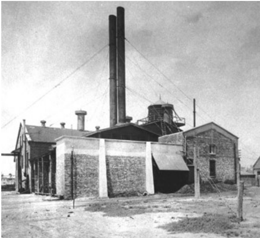
Figure 3: Historical picture of the Key West Diesel Plant facility.
