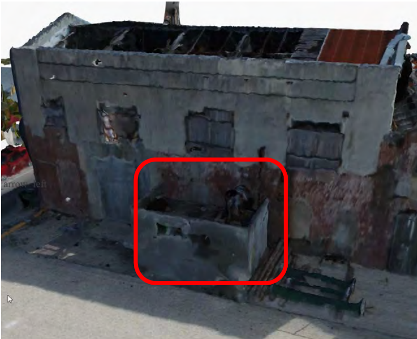
Figure D2: Building 5 from the North East.
