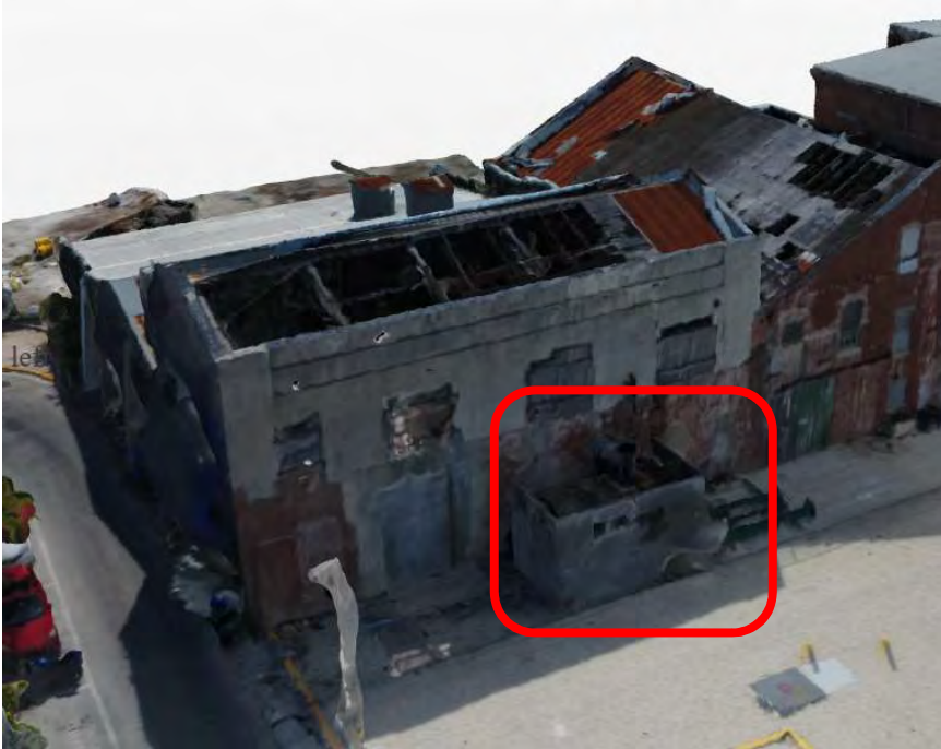
Figure D1: Building 5 from the South East.
