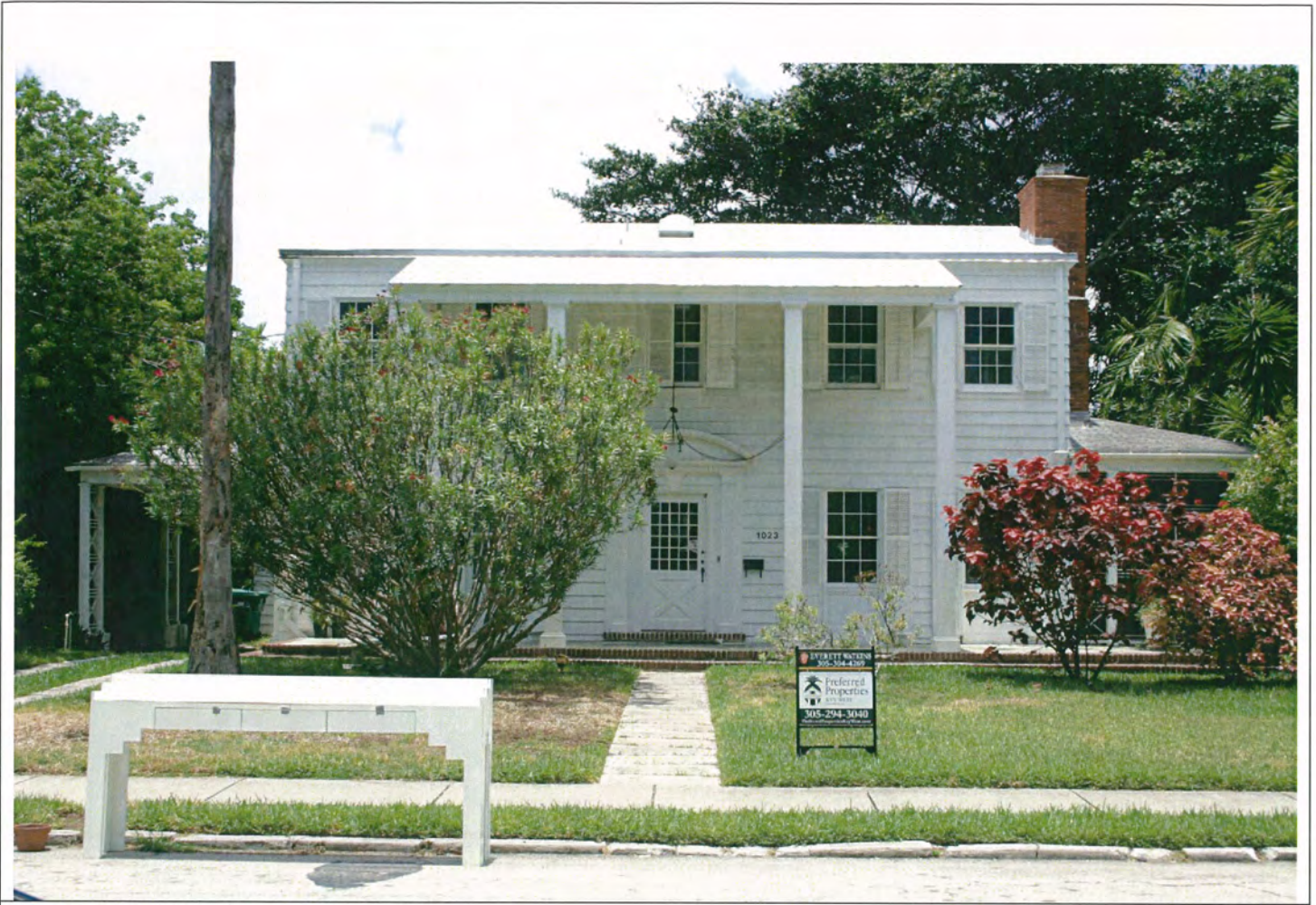
1. 1023 Johnson Street. View from the street.
