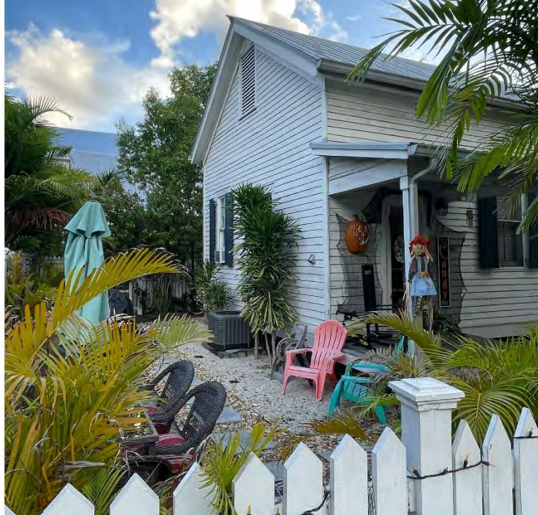
805 Truman Avenue – adjacent to subject site (south).
