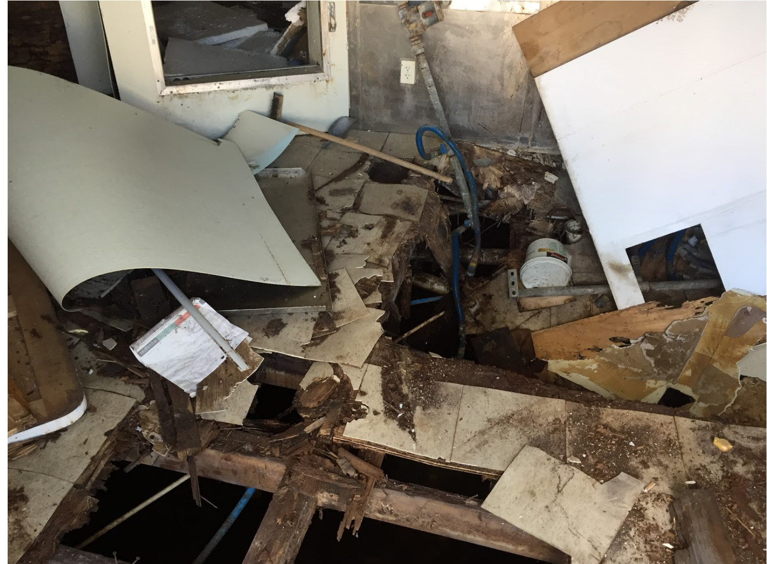
INTERIOR REMOVE DETERIORATED FLOORING AND REPLACE
