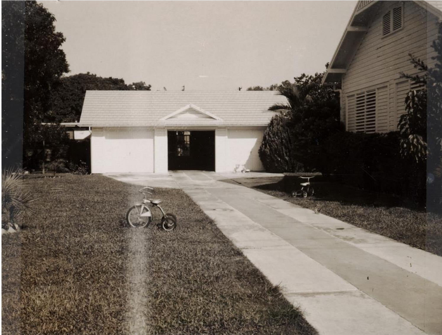
#1021 Washington Street garage circa 1965. Monroe County Library
