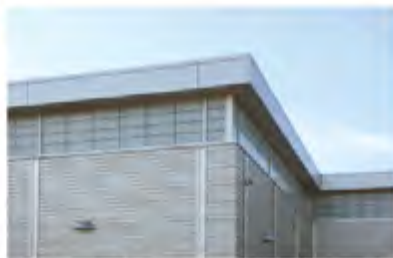
Ivy Tech Community College, Ft. Wayne, IN, MSKTD Architects
