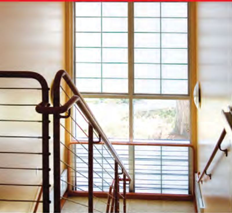
U. of MI Payne Family Native American Center, Miscook, MI, ASF Architects
