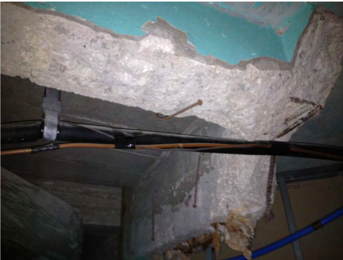
Note wall below beam has been removed and rebar cut
