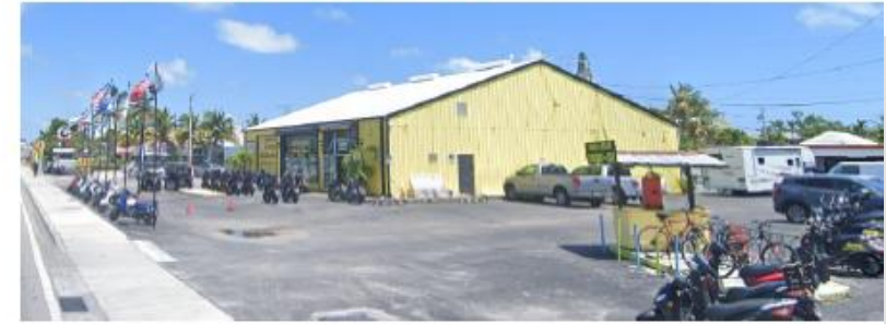
1910 N. ROOSEVELT BLVD. (TO BE DEMOLISHED)
