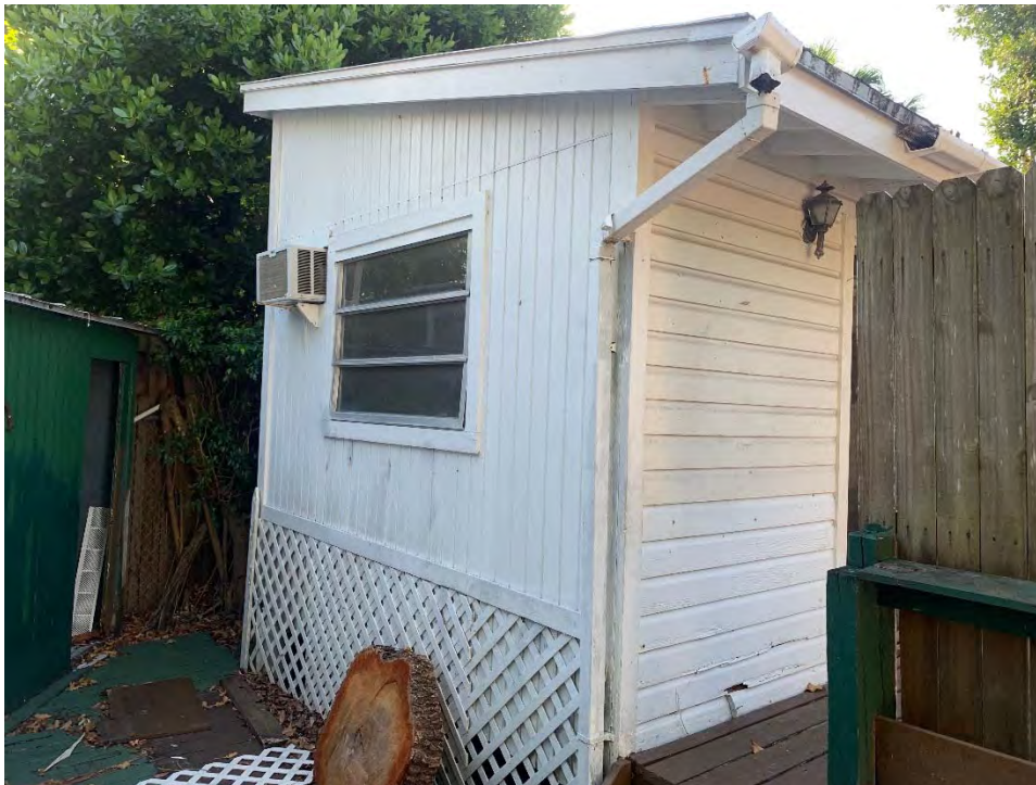
REAR OF PROPERTY LOOKIING TOWARD FRONT
