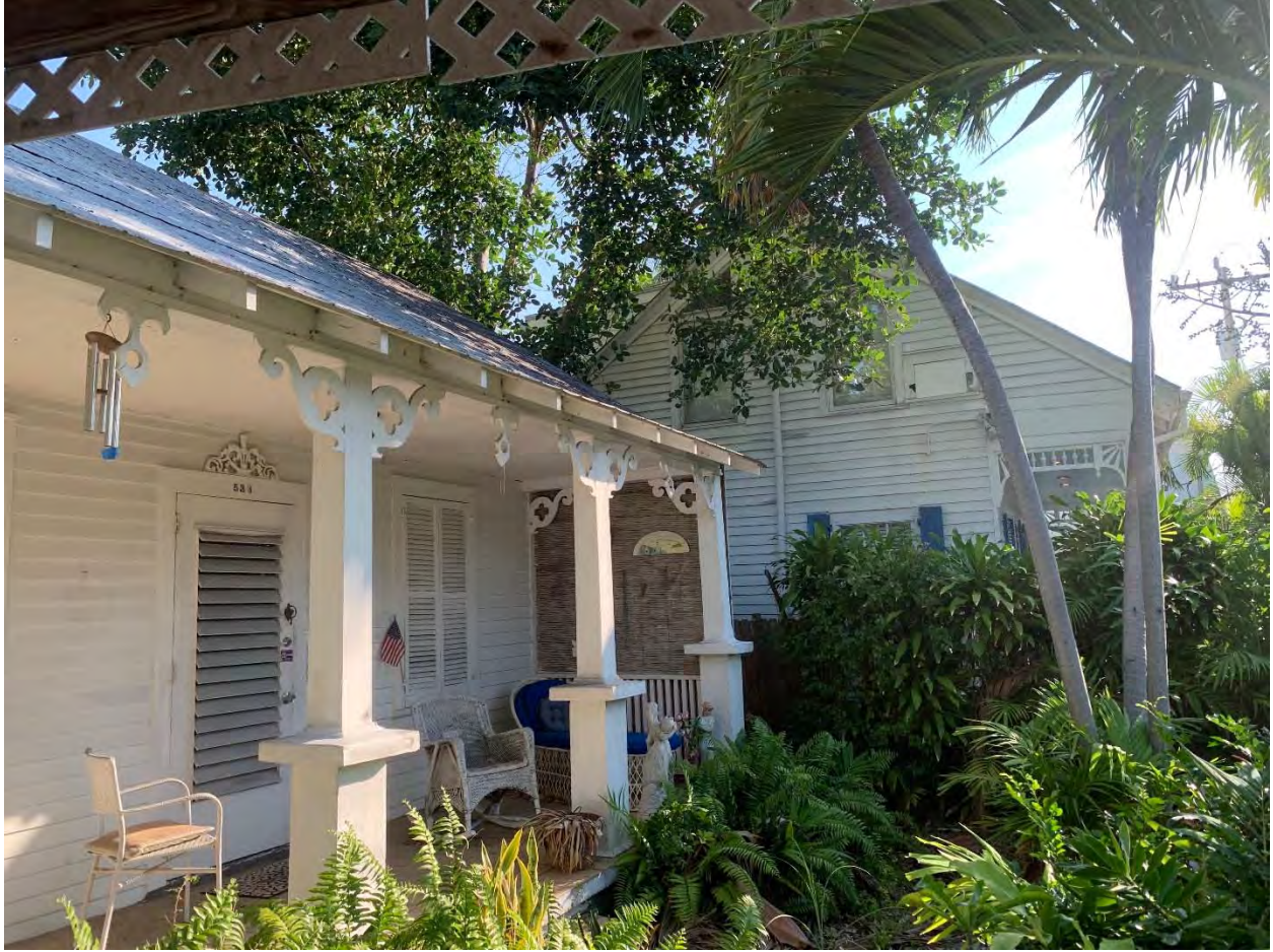
NEIGHBOR TO EAST
