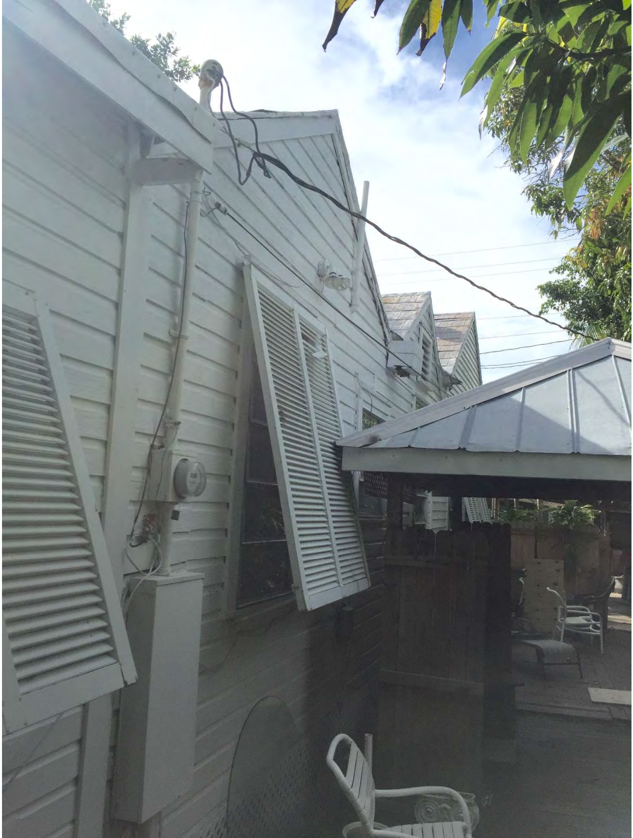
MAIN ROOF (RIGHT) AND 2 SAWTOOTH ADDITIONS (LEFT) TO REMAIN
