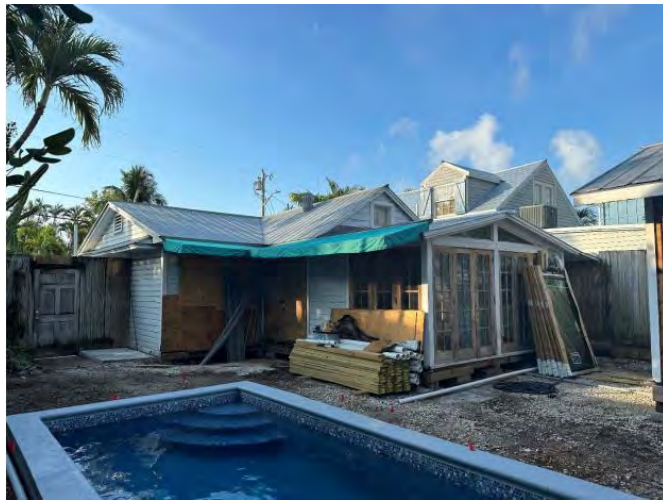
Existing Rear of Historic Structure
