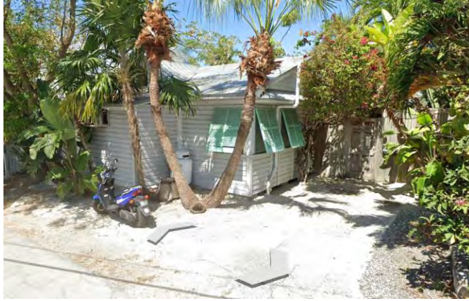
Existing Front of Historic Structure
