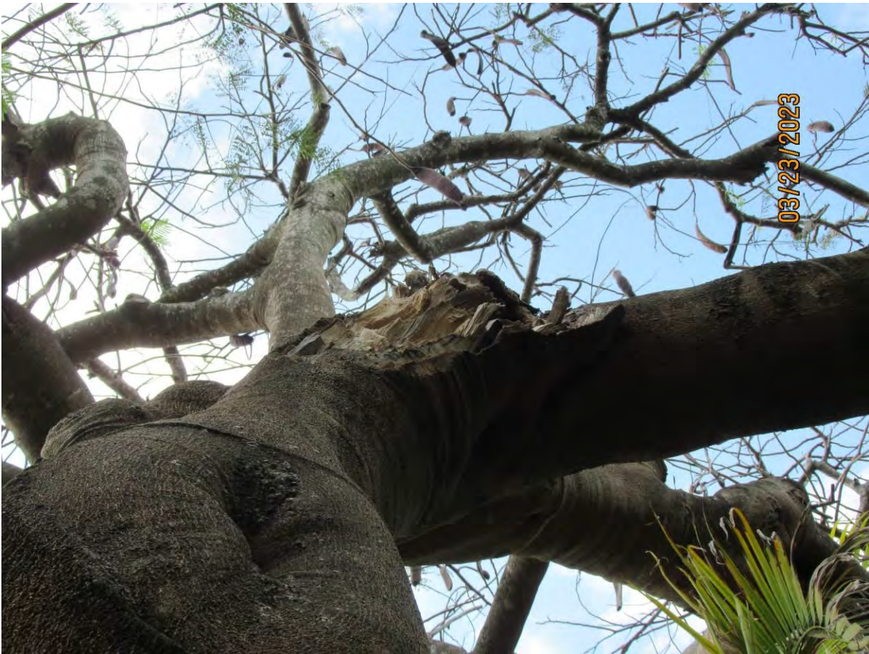
Two photos of canopy branch break 1.
