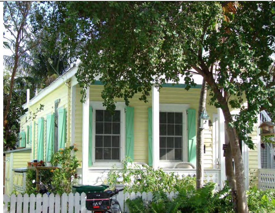
PHOTO 2- 1404 Olivia House: View from Street NE
