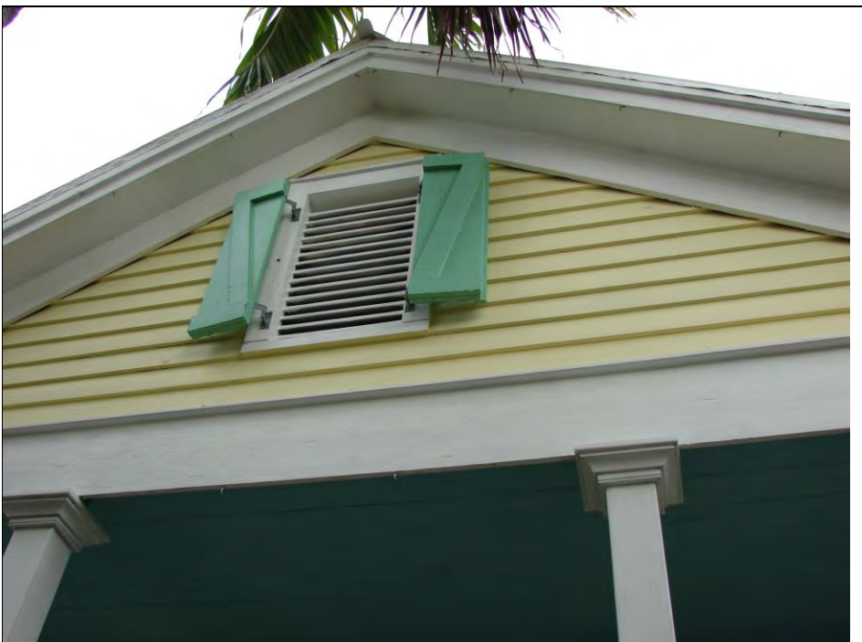
PHOTO 7- 1404 Olivia House: View from Street - Gable
