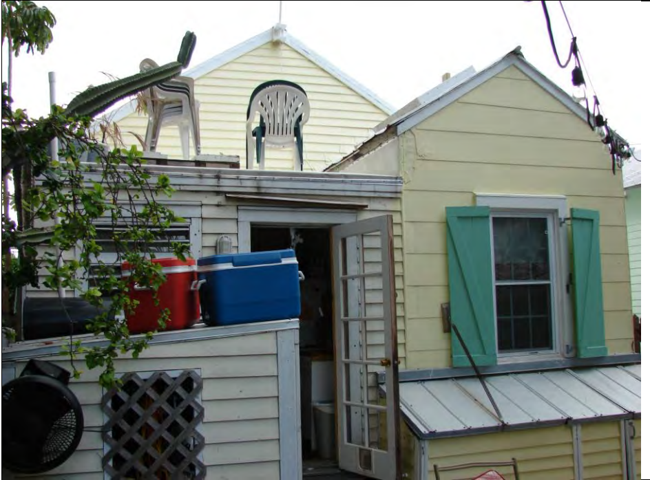
PHOTO 6- 1404 Olivia House: Sheds to be Rebuilt
