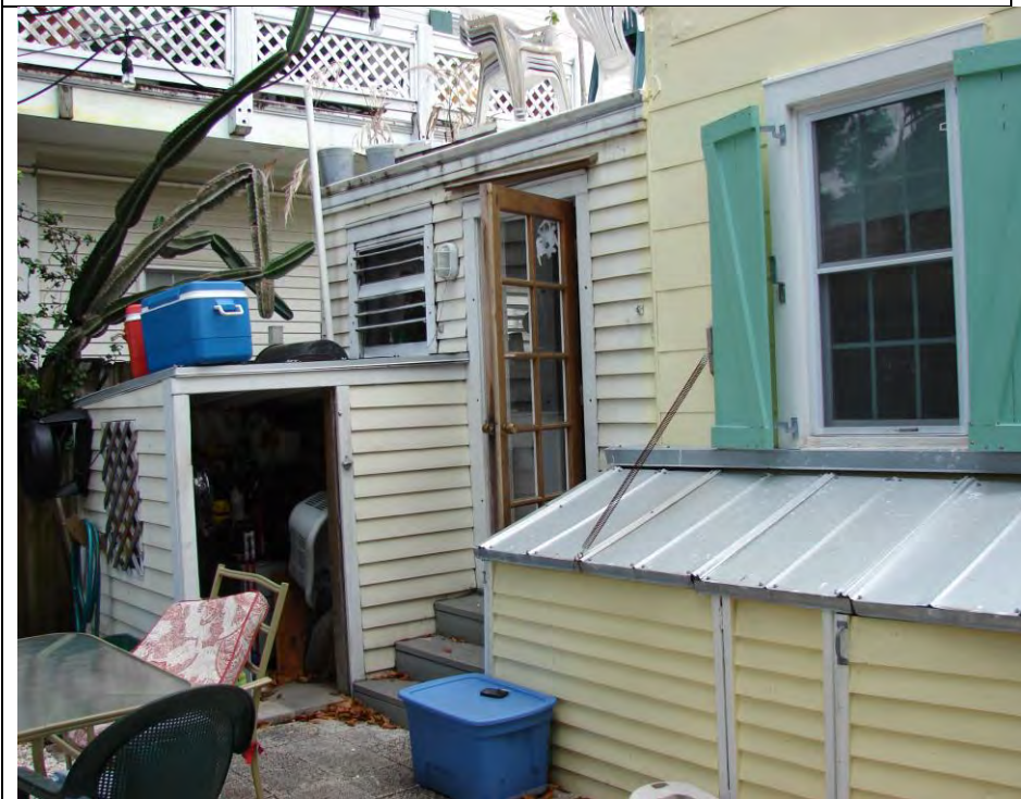
PHOTO 5- 1404 Olivia House: Sheds to be Replaced
