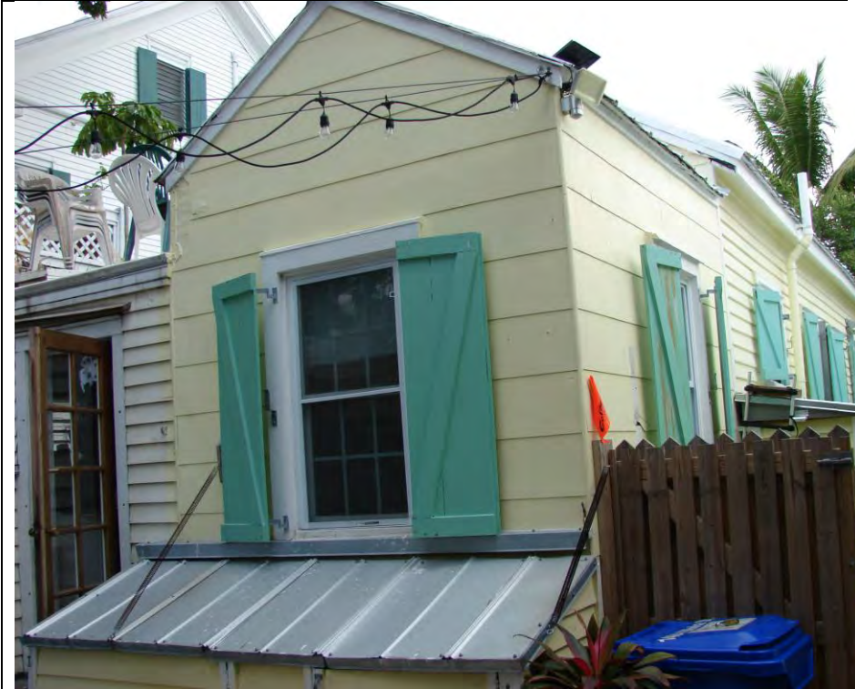
PHOTO 4- 1404 Olivia House: View from Rear –Existing
