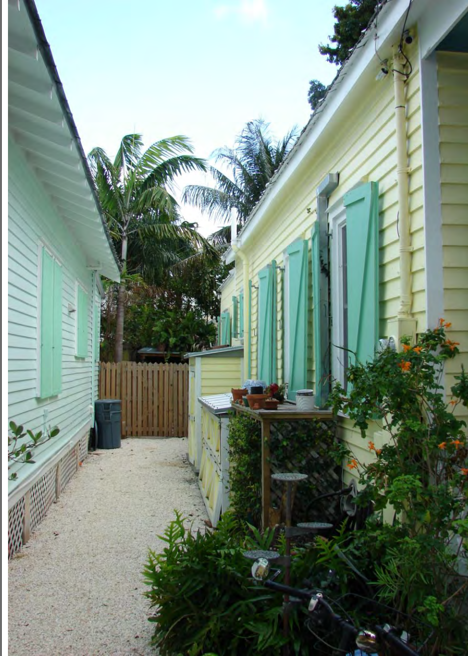
PHOTO 3- 1404 Olivia House: View from side yard
