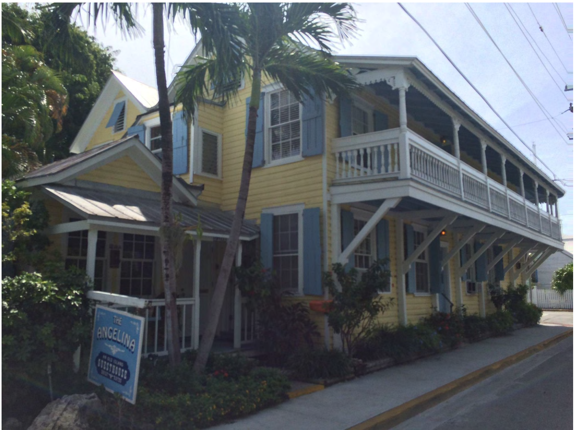
Building located at the corner of Angela Street and Thomas Street
