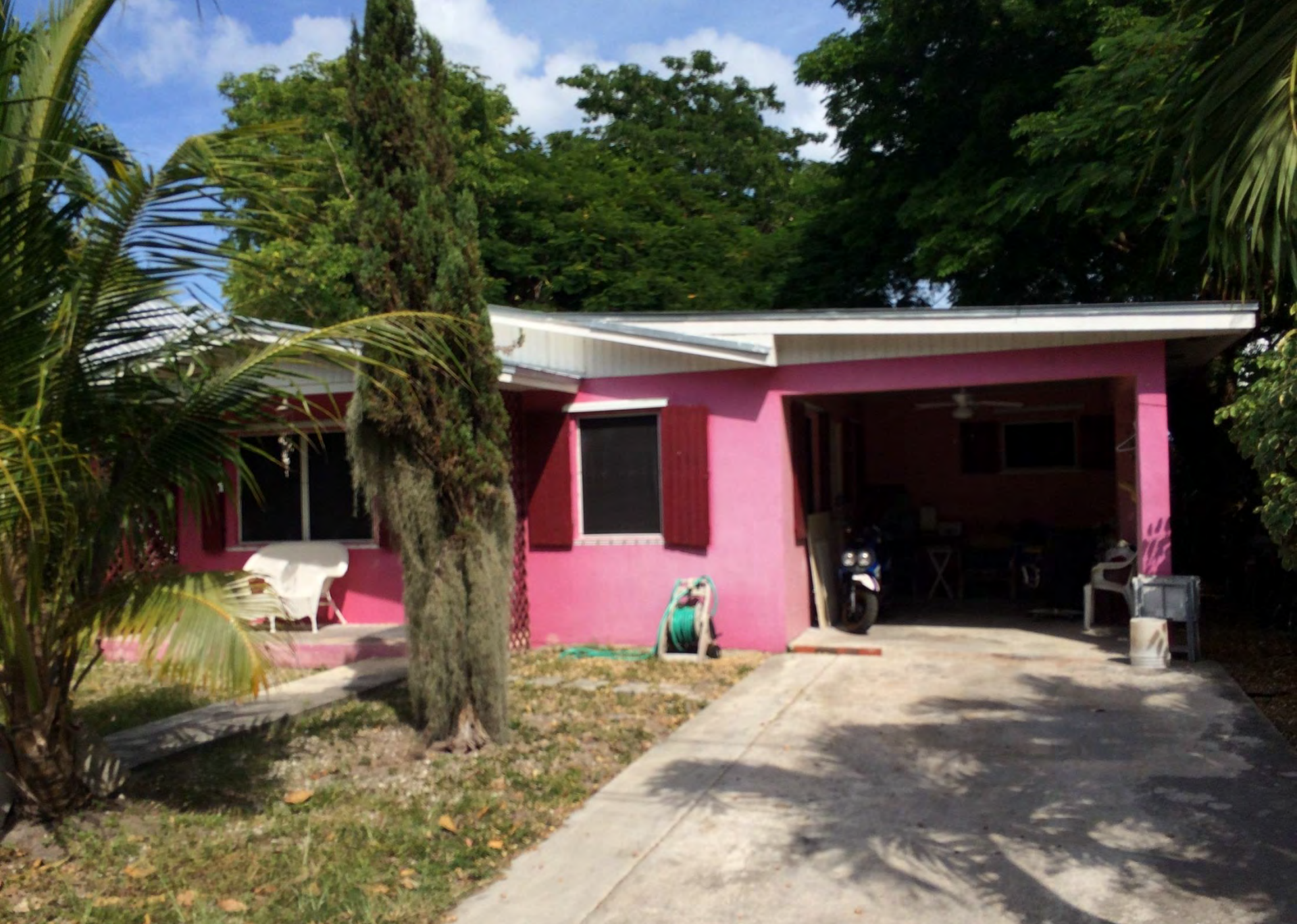
619 Mickens Lane – the neighboring structure on Mickens Lane
