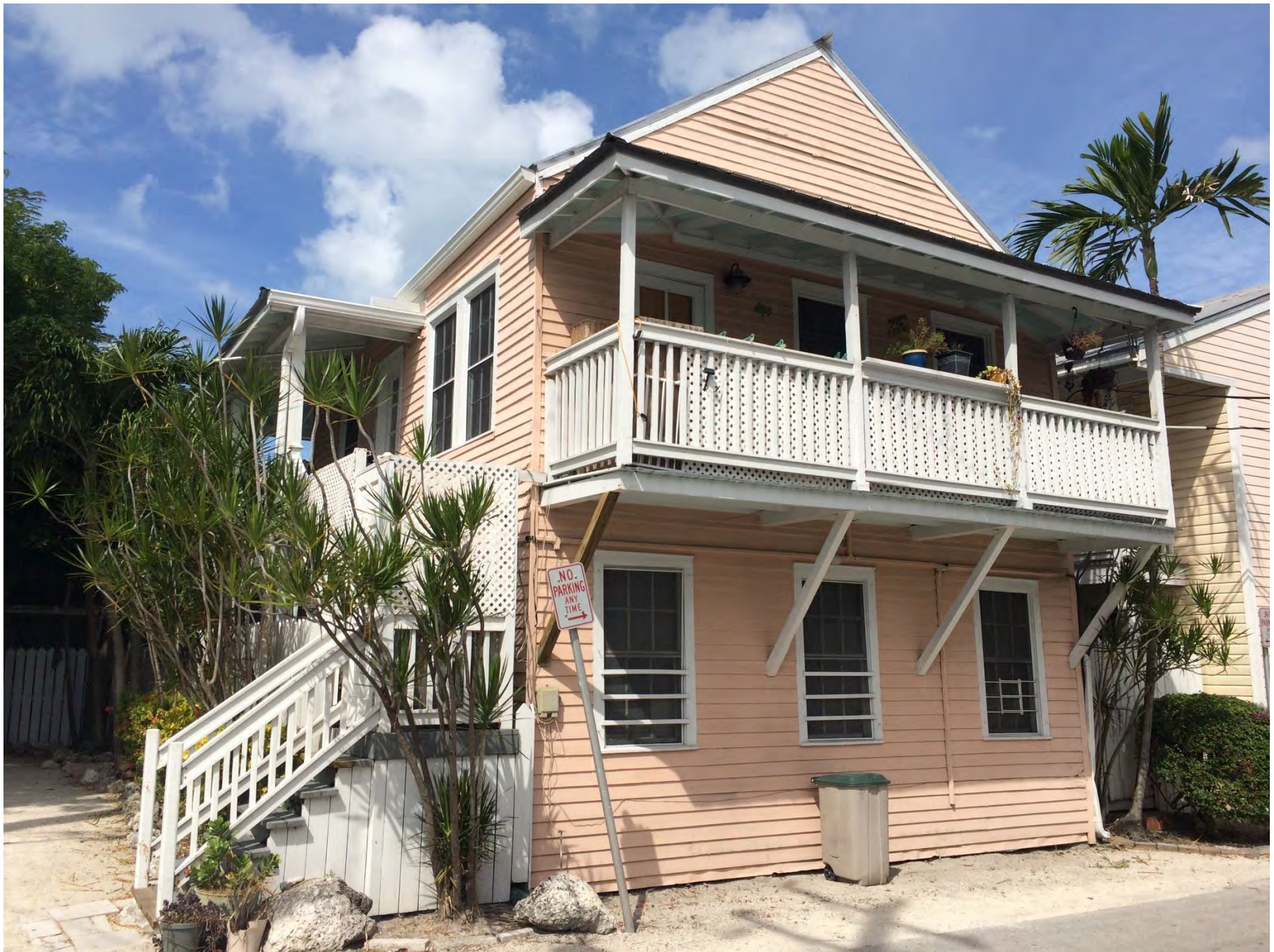
Part of 632 Whitehead Street
