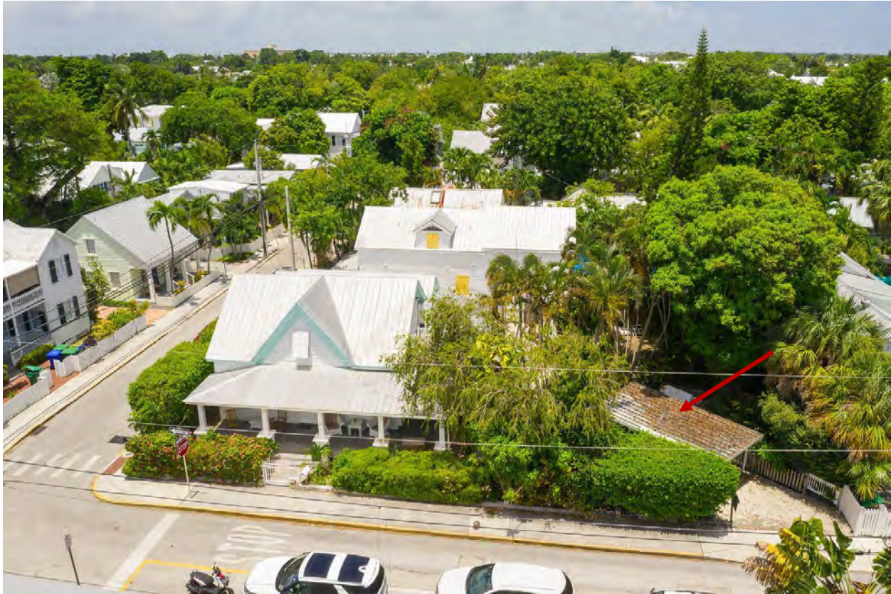
Aerial photograph of the site under review showing the non-historic carport.
