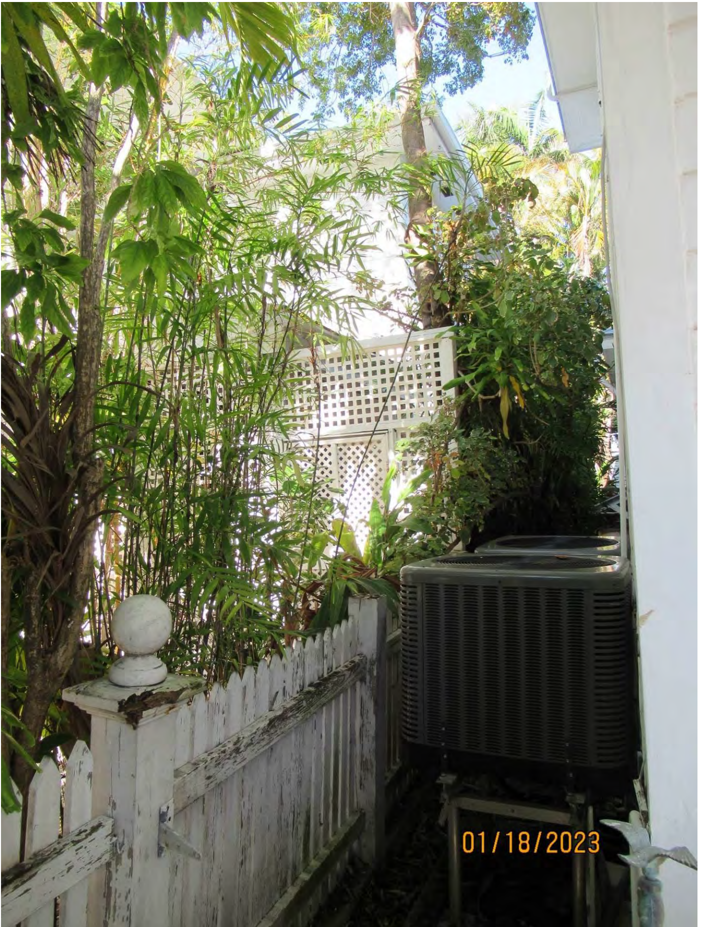
Photo of tree trunk and its location between the two buildings.
