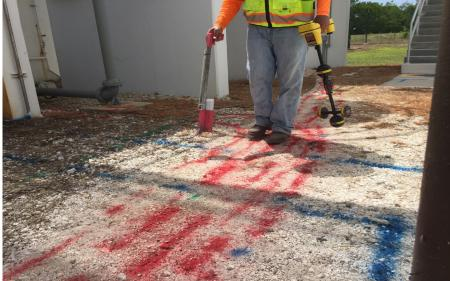
Longitude Surveyors (LS) performed a full Topographic Survey and Subsurface Utility Engineering services as described below:
