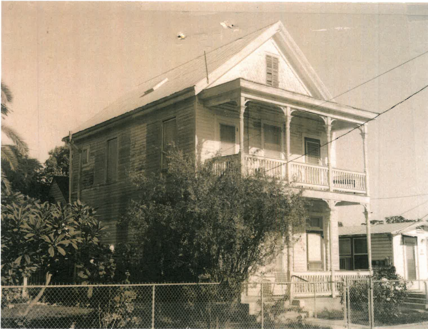
#803-805 Olivia Street Property Appraisers office. Building to the right side is the structure in question for this application. Monroe County Library
