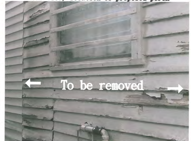
Southeast view of rear shed addition
