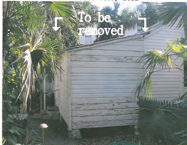
Southwest view of rear shed addition
