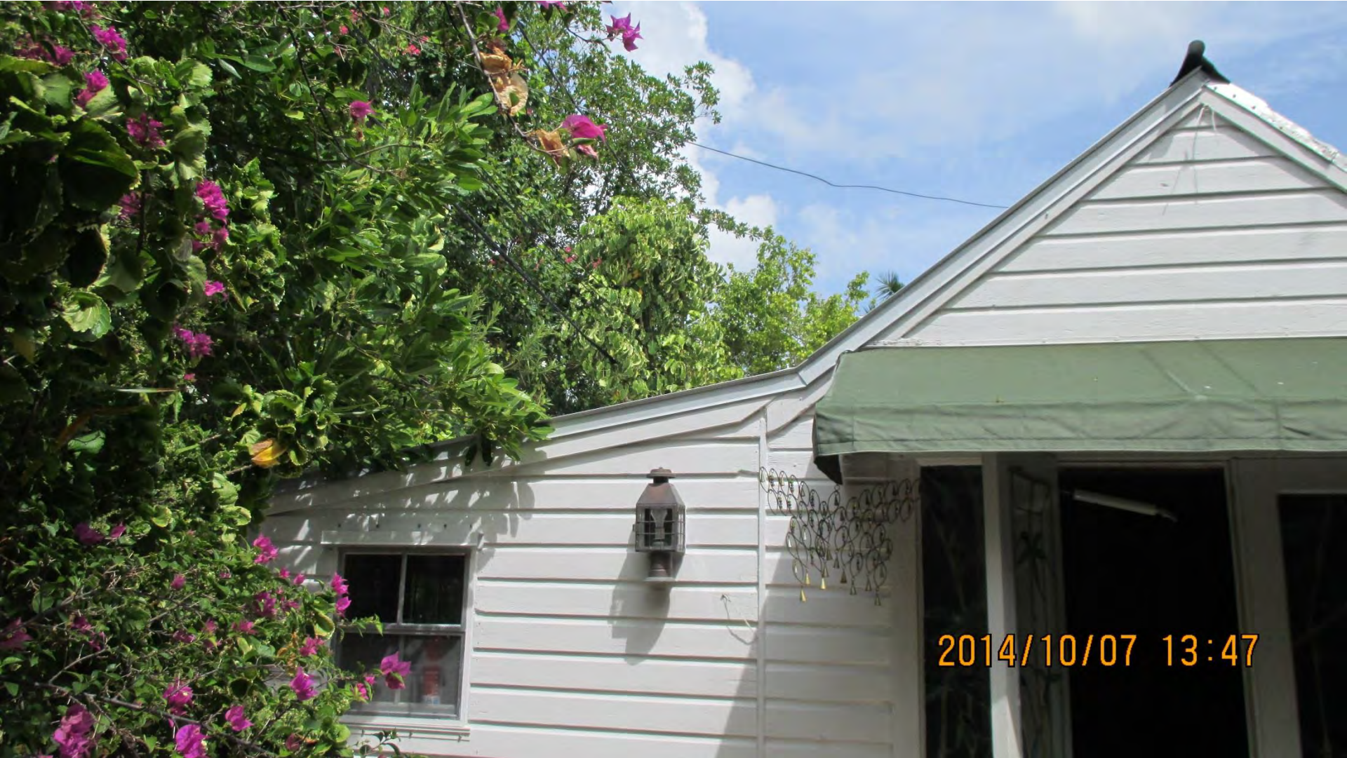
Rear gable roof that has the hip front.
