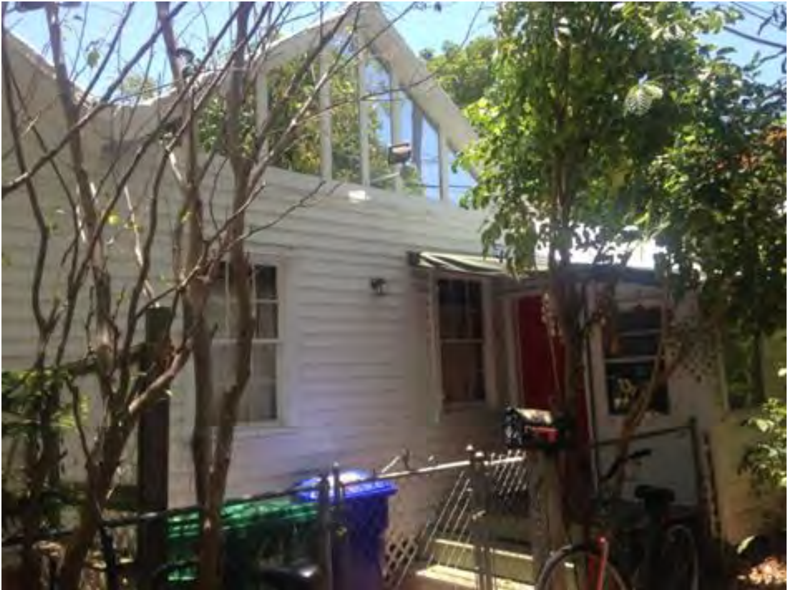
Inappropriate clerestory windows to be removed.
