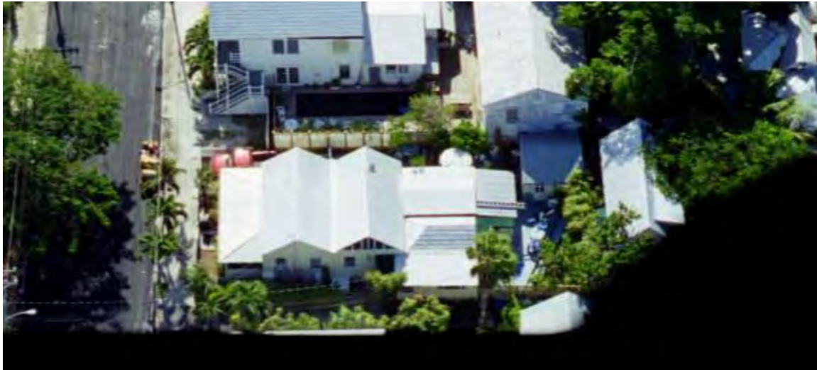
2000 Bird's Eye photo showing the different roof forms.
