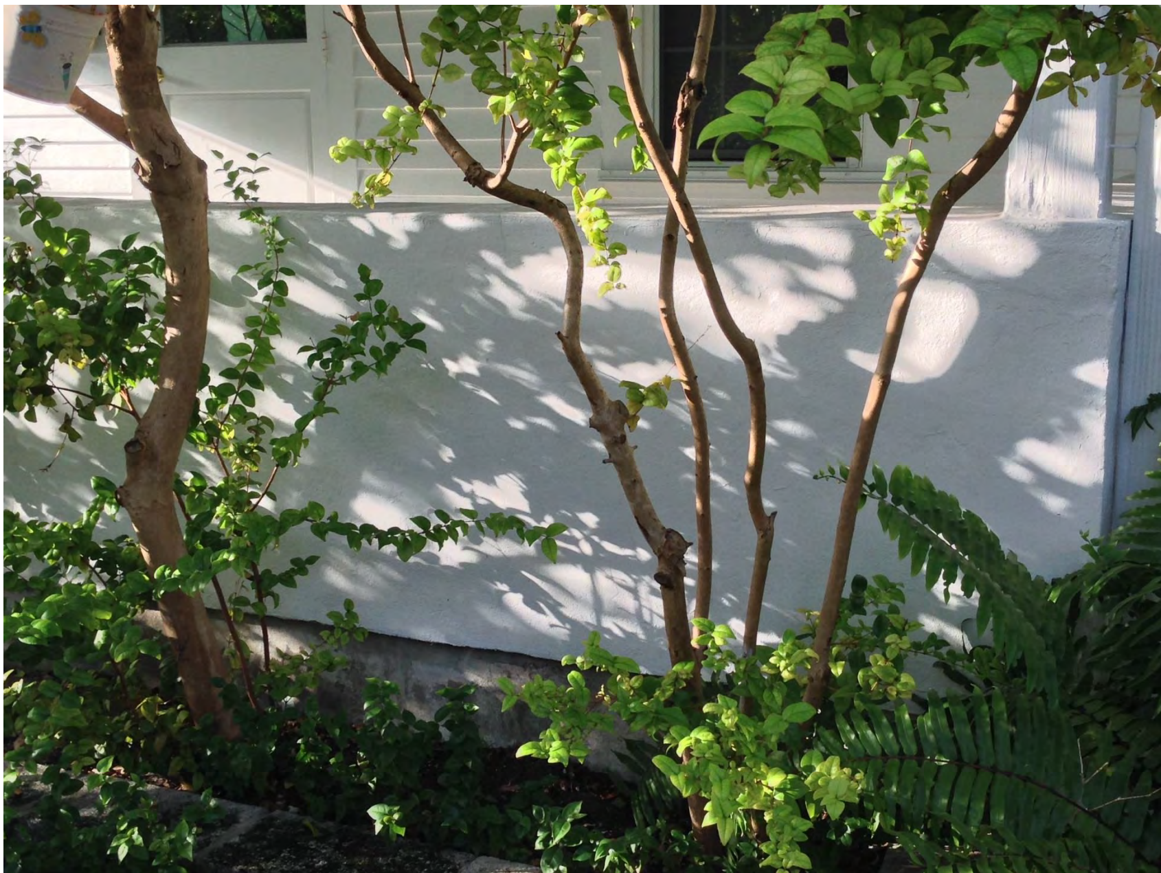
Close up of concrete porch wall.
