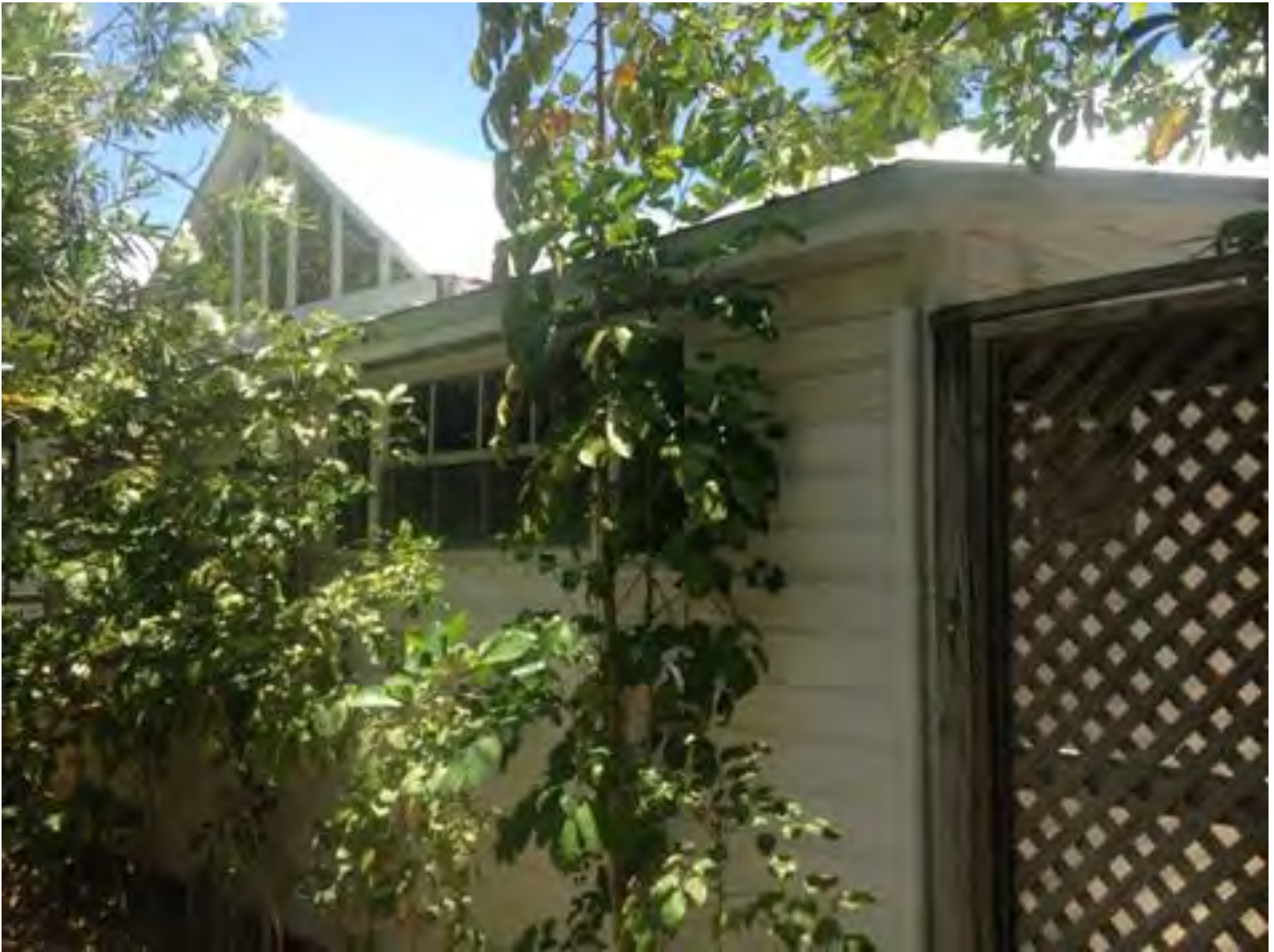
Another view of the south side of the house. Rear of the shed roof section that will be moved off city right-of-way.
