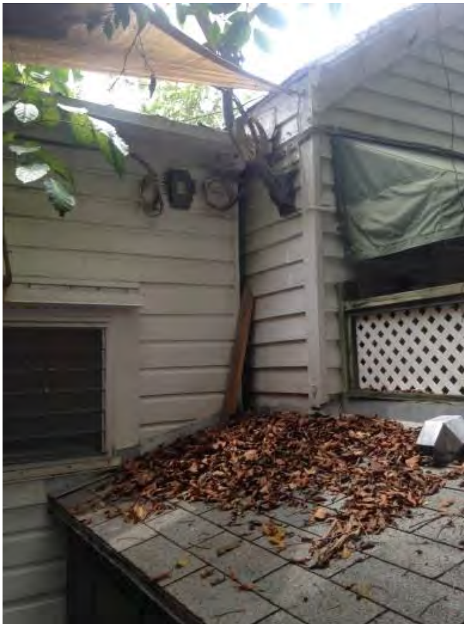
Close up of the connection between the second sawtooth roof and rear gable roof on south side of house. Even though Sanborn maps do not show this as an addition, it looks like one.
