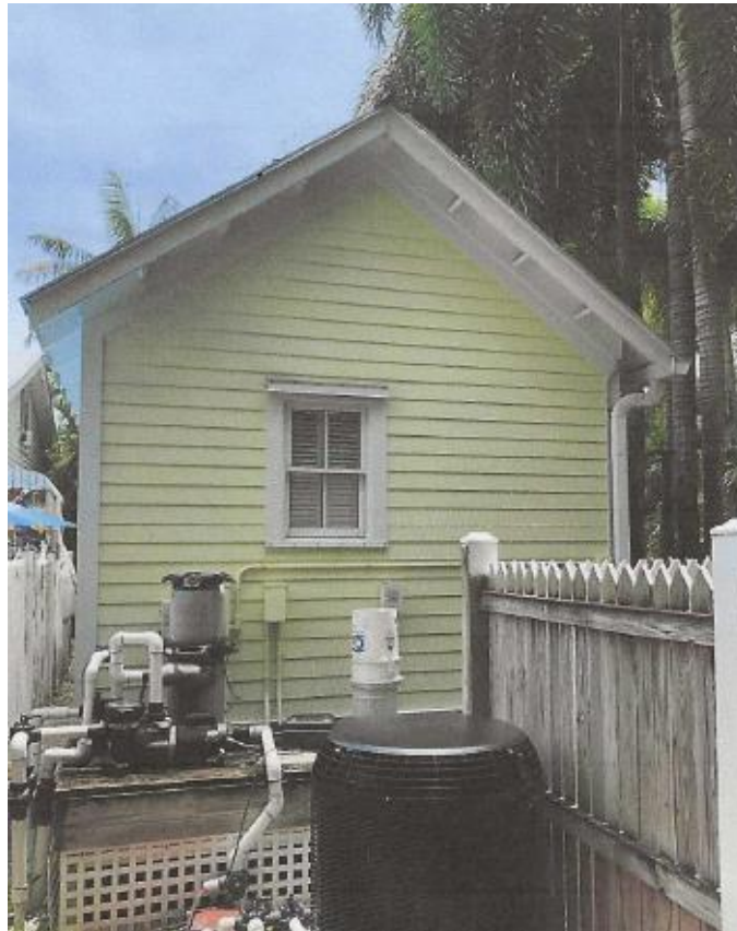
Rear of property looking south at existing addition.
