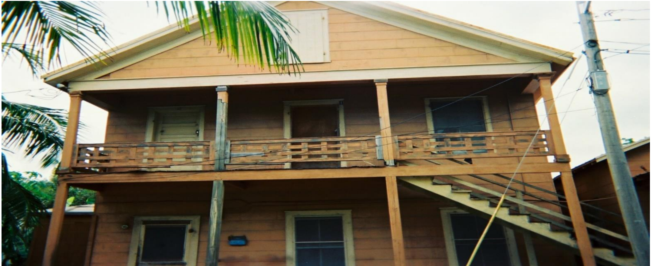
PRE-CONSTRUCTION TWO-STORY MAIN BUILDING
