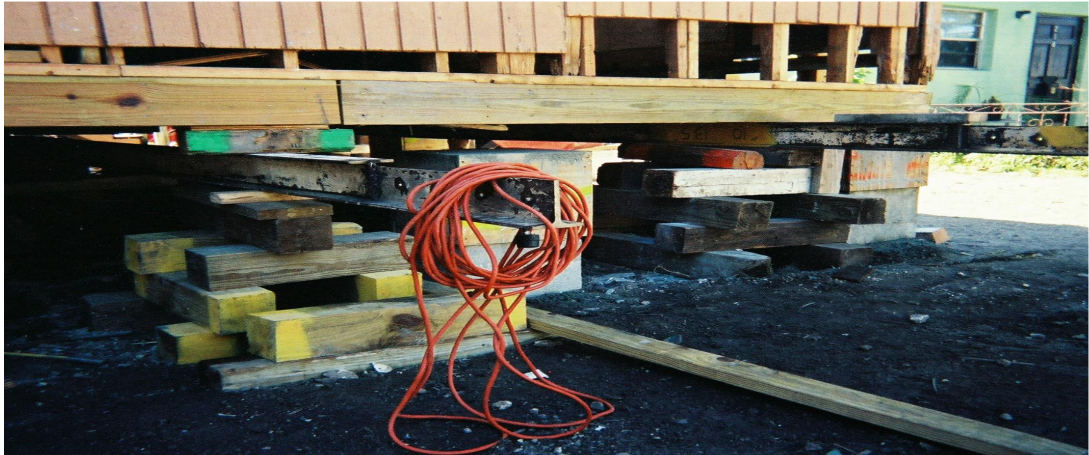
BUILDING RAISE SHOWING HEIGHT OF FOUNDATION COLUMN REBUILD
