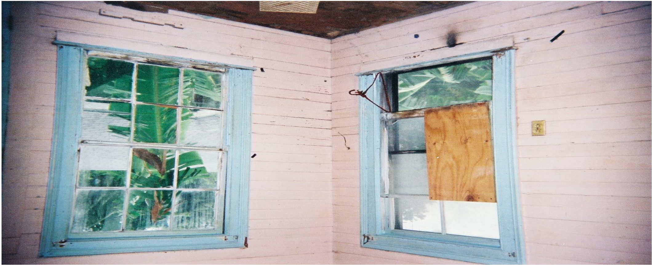
NORTHEAST UNIT CORNER DADE COUNTY PINE
