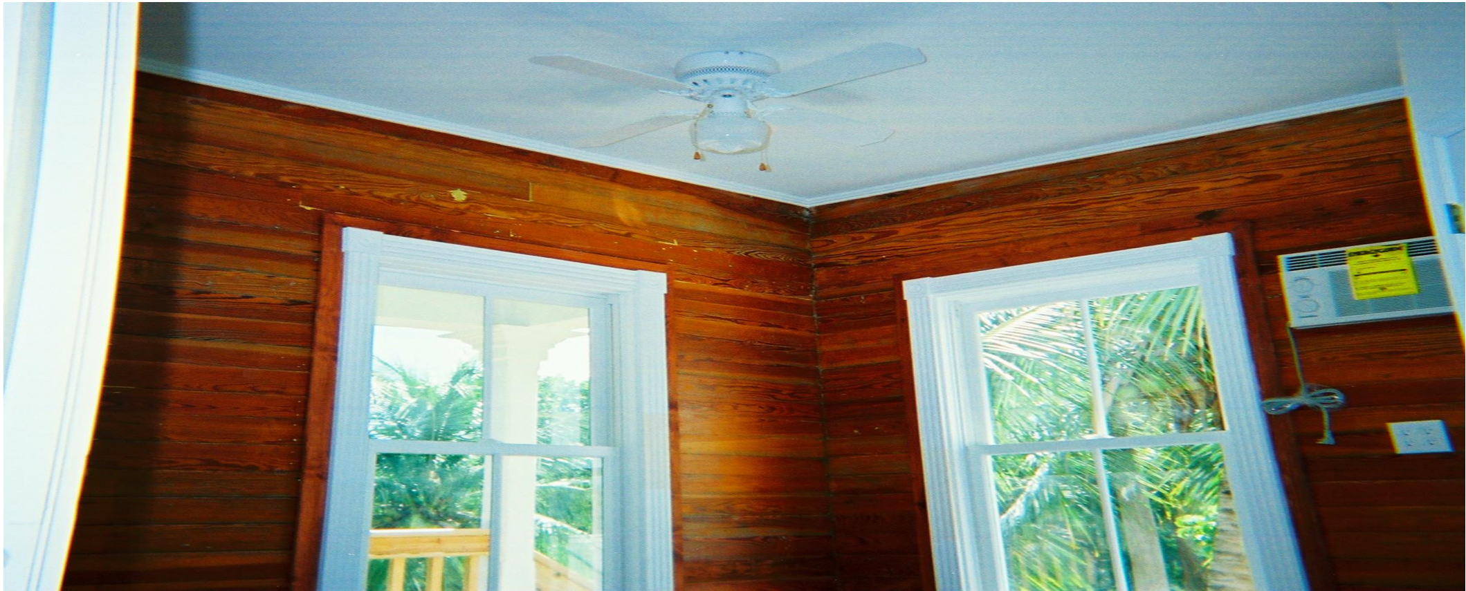
NORTHEAST UNIT CORNER DADE COUNTY PINE
