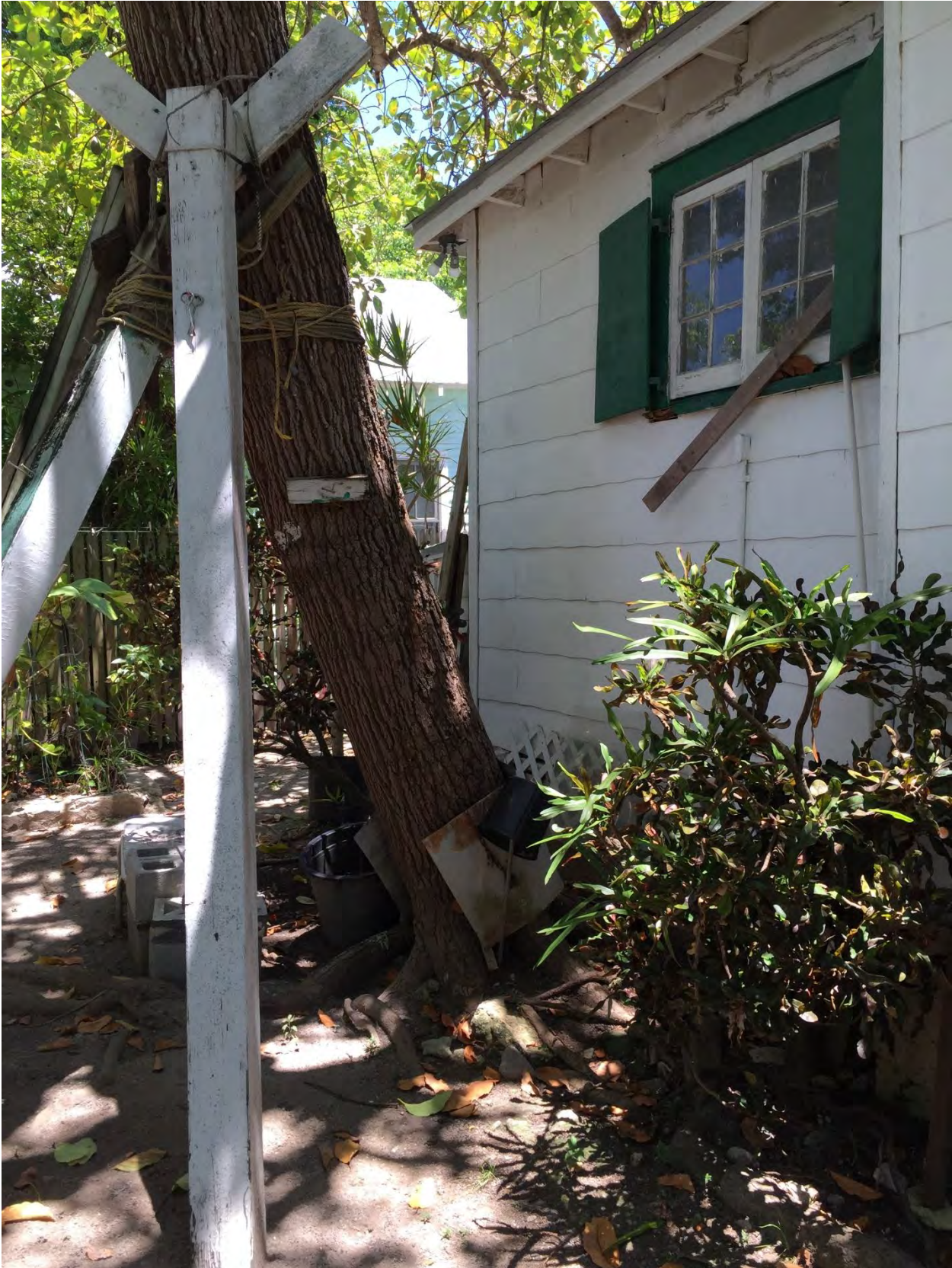
Rear portion to be removed
