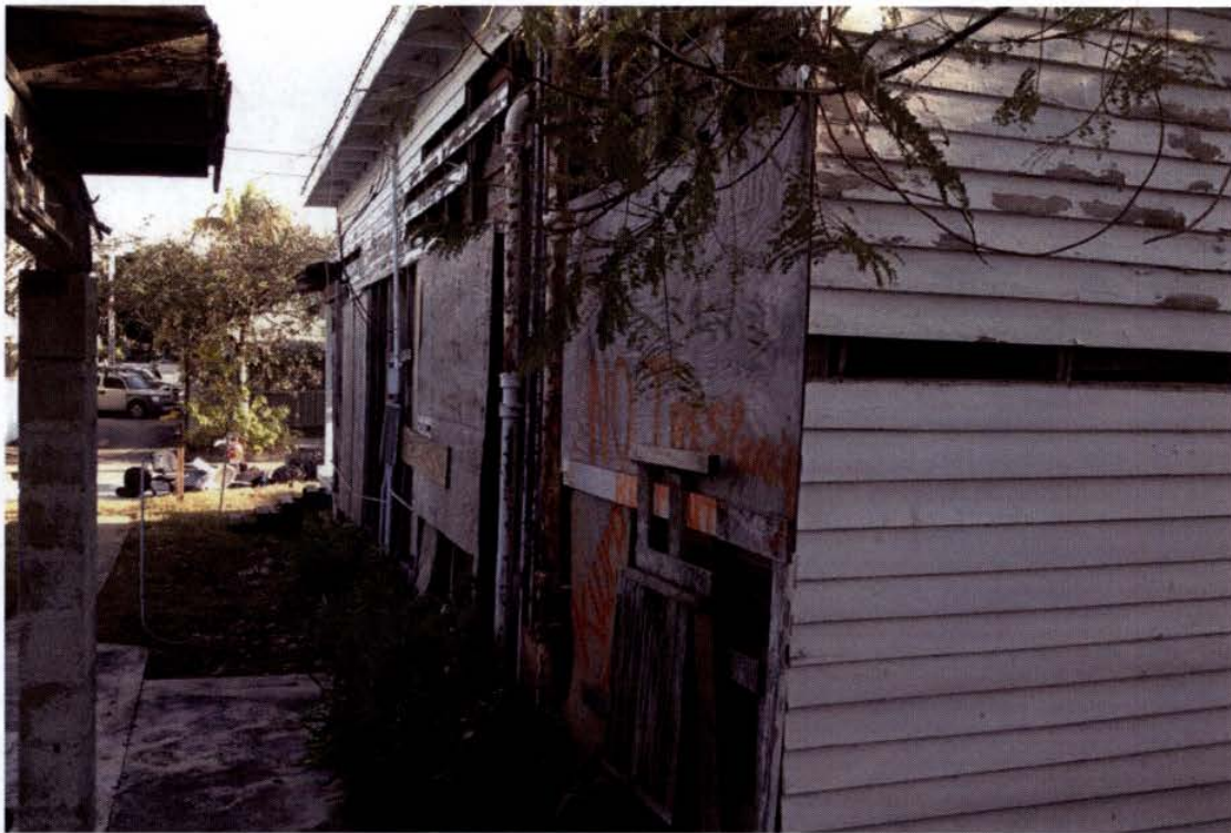
NORTHEAST ELEVATION LOOKING TOWARDS VIRGINIA ST.
