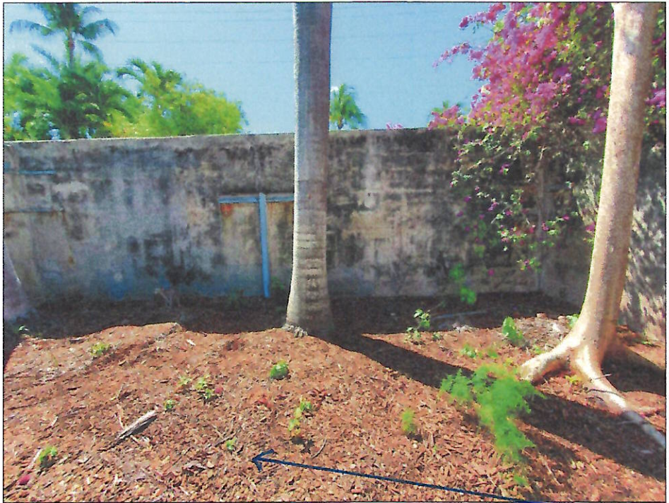
LOOKING GSW - REAR YARD - POOL HOUSE
