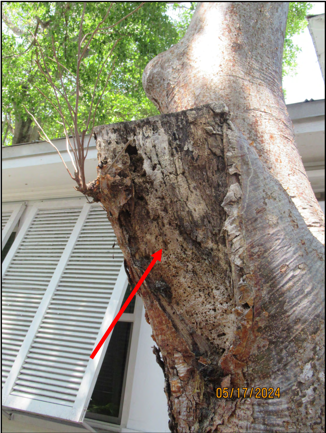
GL1: Termite and multiple species of woodboring beetle damage in wound; suspect Ambrosia beetle, suspect Flatheaded borer, suspect termite infestation.
