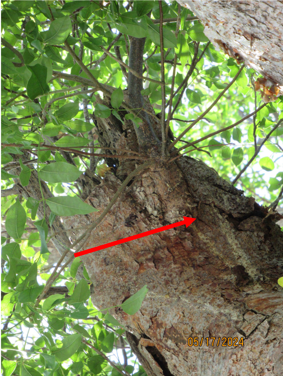
Aerial termite damage
