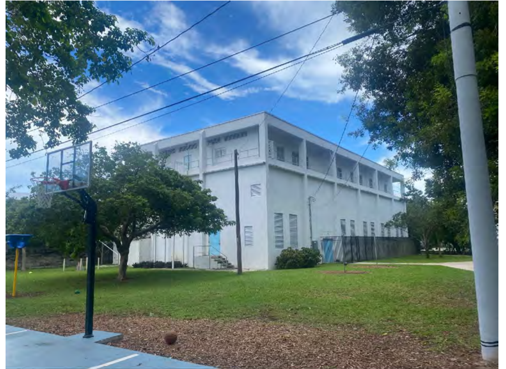
700 TRUMAN AVE. SIDE VIEW (LEFT SIDE OF BUILDING)
