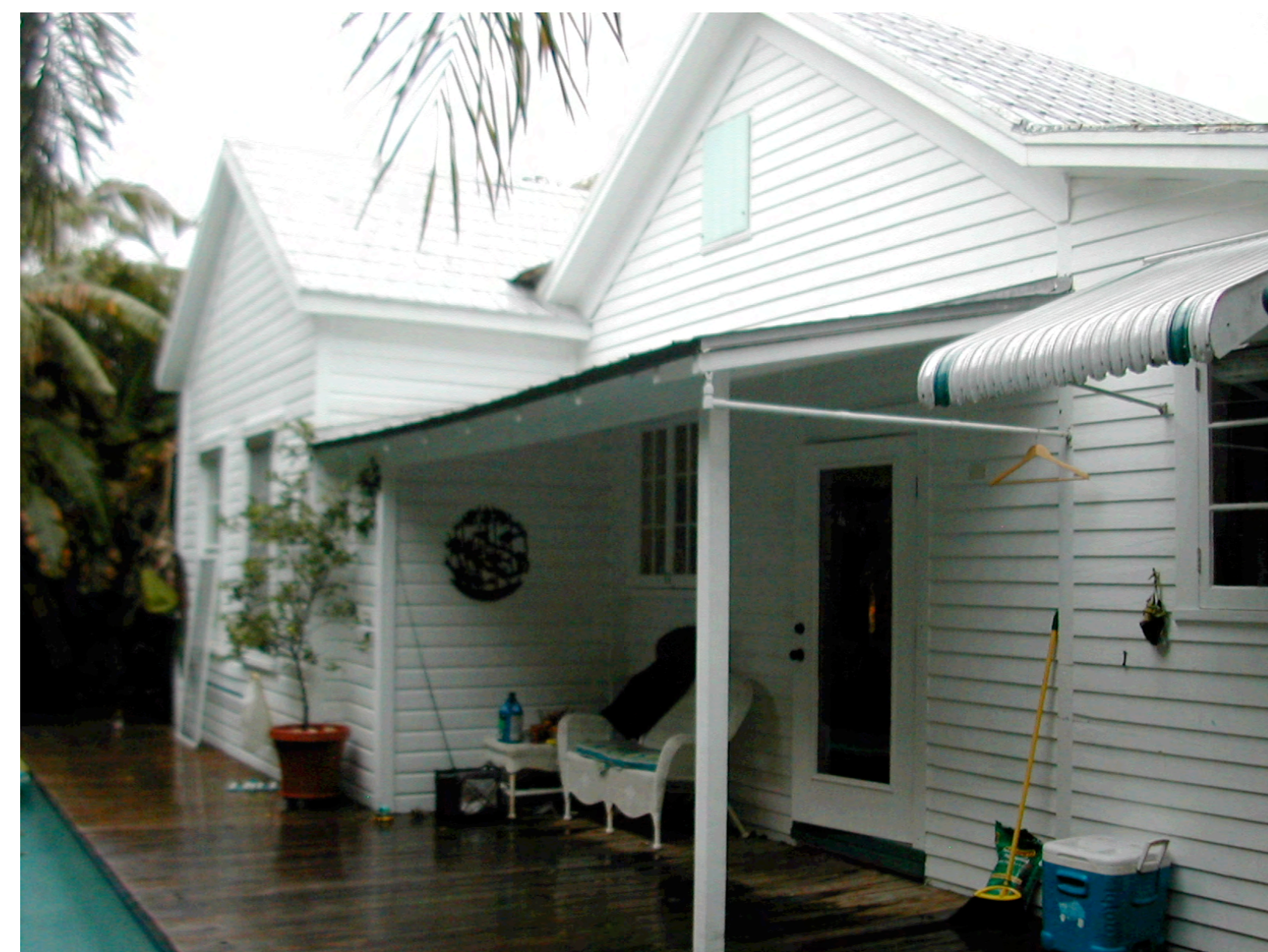
VIEW OF REAR SIDE OF HOUSE SHOWING EXISTING DOOR, WINDOW, AND SHED ROOF TO BE REMOVED
