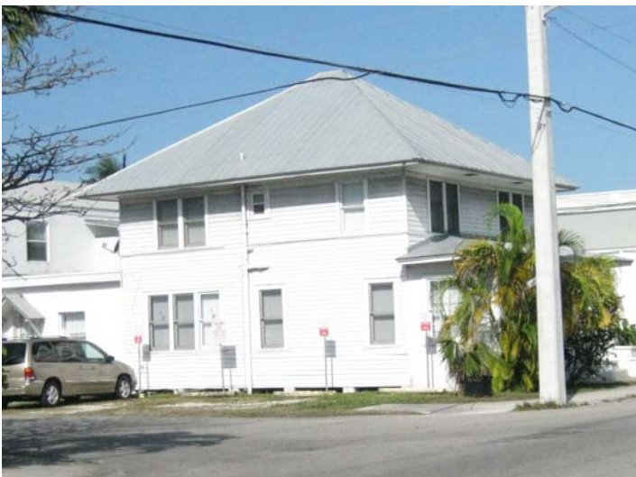
Another Foursquare house on White Street
