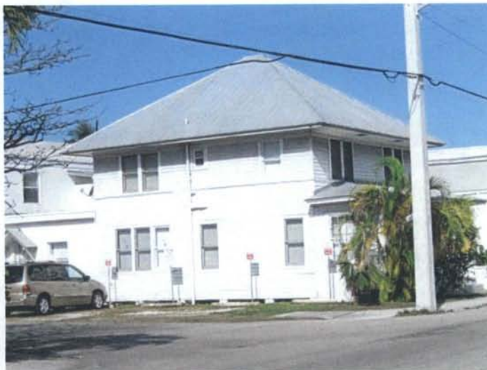
Another Foursquare house on White Street
