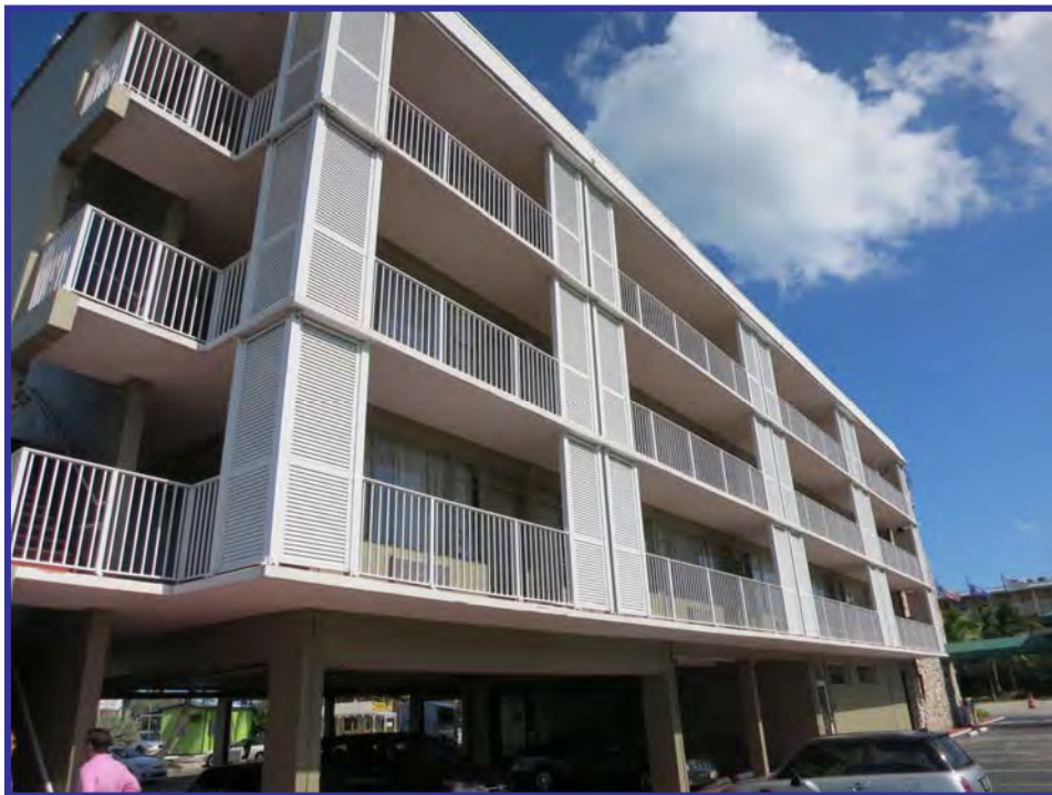
View of the 4-story building's south elevation
