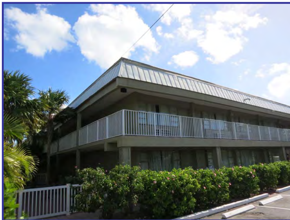
View of the northwest corner of the 2-story north building
