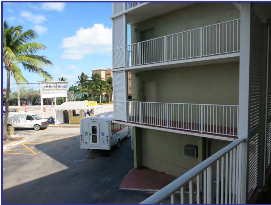
Covered exterior walkways and railings (4-story building)
