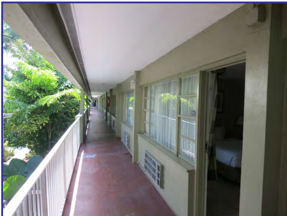
View looking south along the east elevation of the 2-story north building (second floor)
