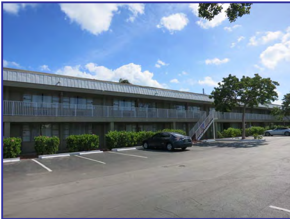
View of the east side of the 2-story north building
