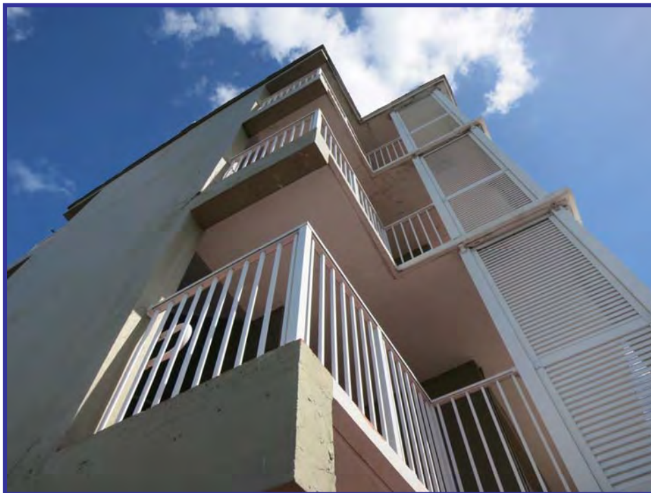
View of the cantilevered exterior stairway and balcony
