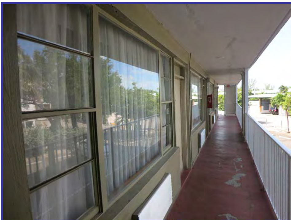
Close-up view of covered exterior walkway (4-story building)
