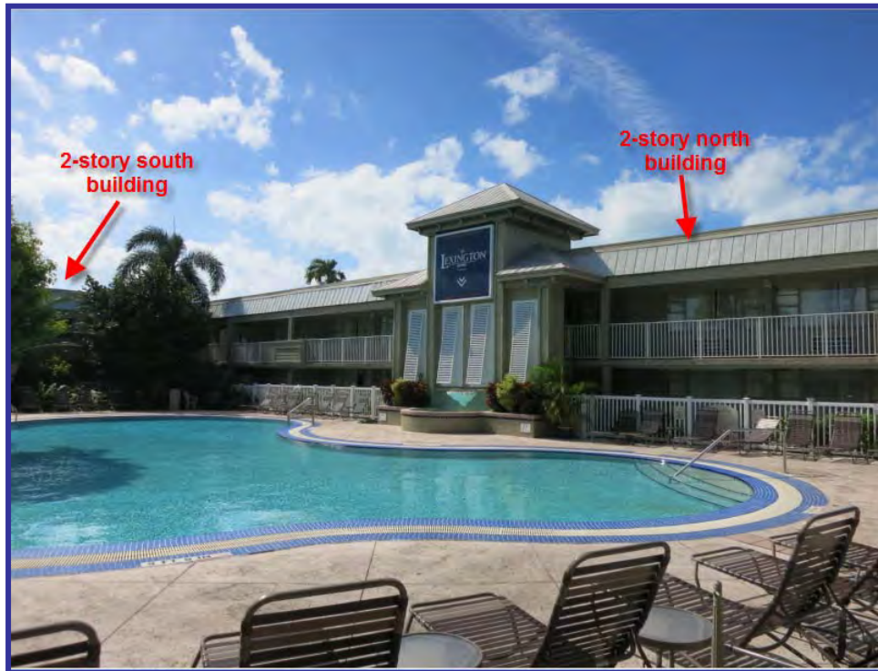
View looking southwest across the pool area
