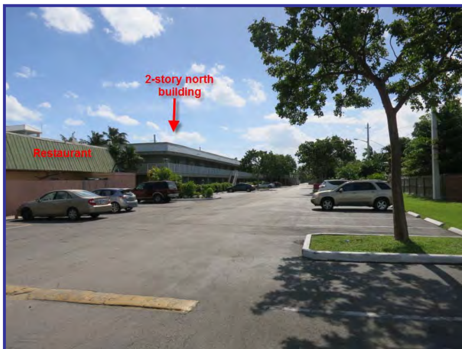
Looking south along the west parking area.
