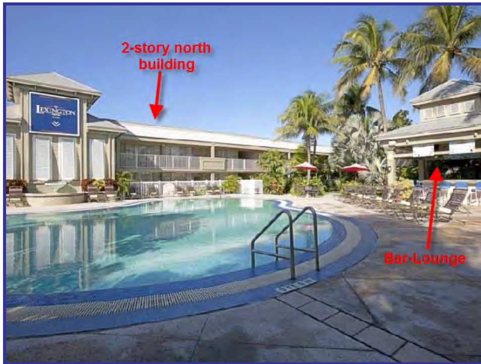
View looking northwest across the pool area
