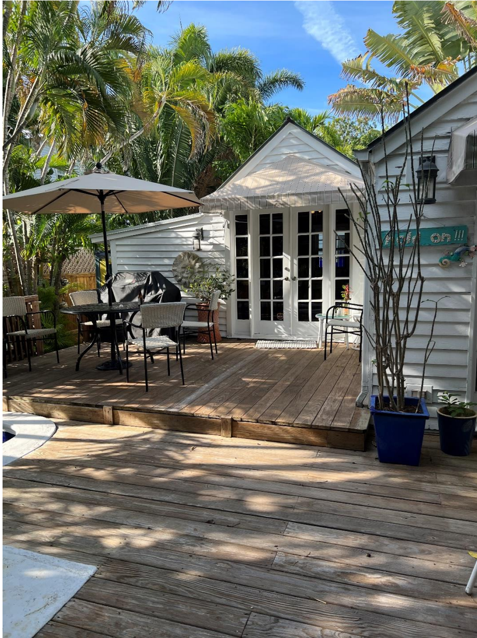
side photo of area of work standing near pool
