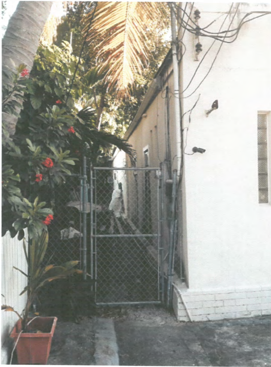
EXISTING CONDITIONS – 1111 MARGARET ST. (NORTH SIDE VIEW)
