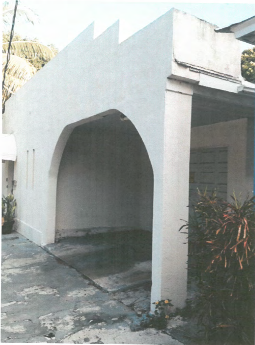
EXISTING CONDITIONS – 1111 MARGARET ST. (PORTICO FROM SOUTH SIDE)
