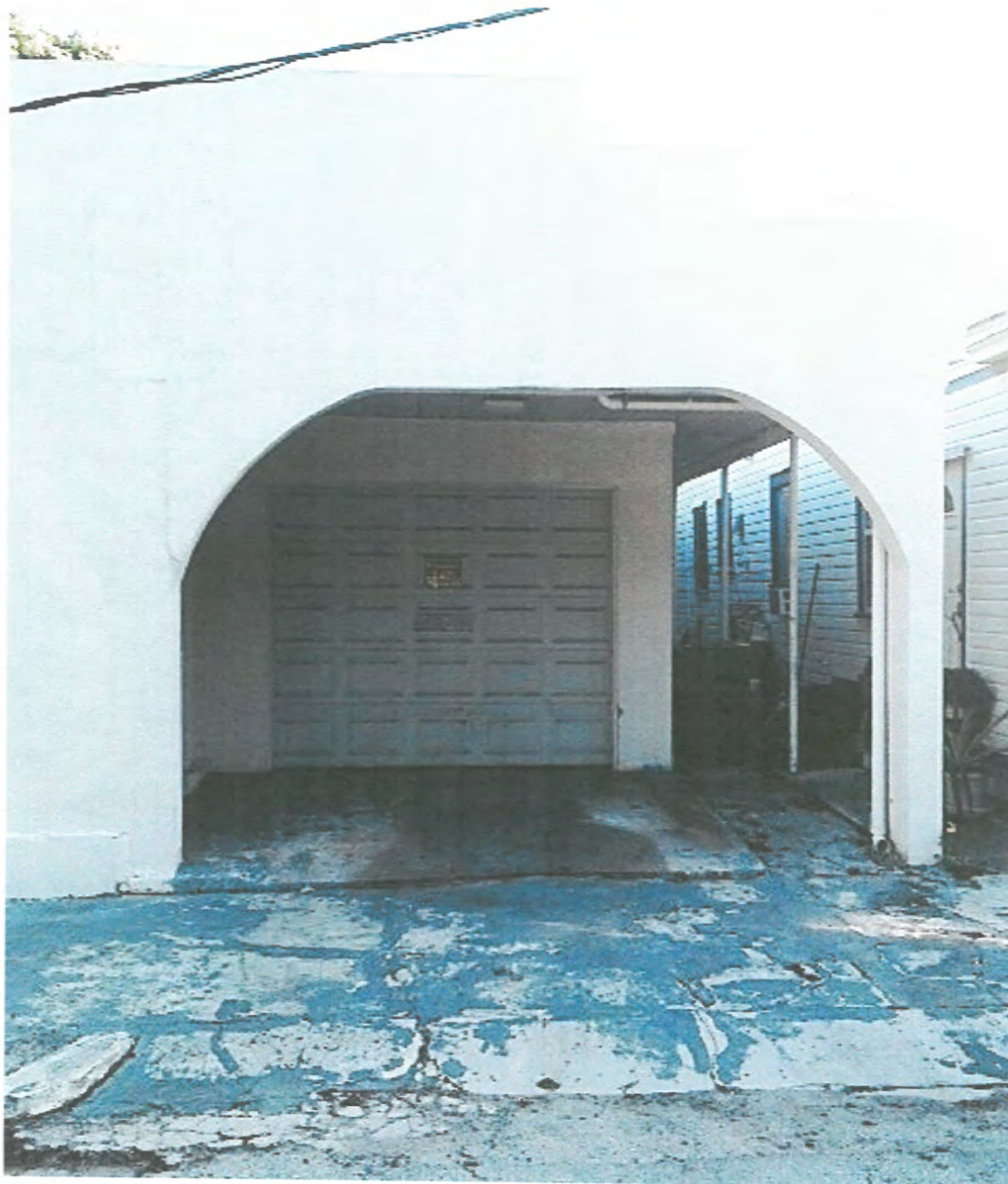
EXISTING CONDITIONS – 1111 MARGARET ST. (PORTICO FROM FRONT)
