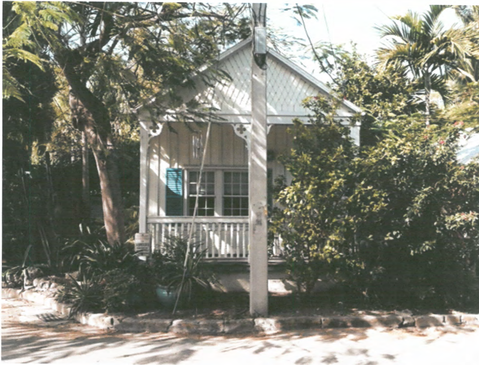
ADJACENT PROPERTIES – 1111 (SECOND FROM NORTH)
