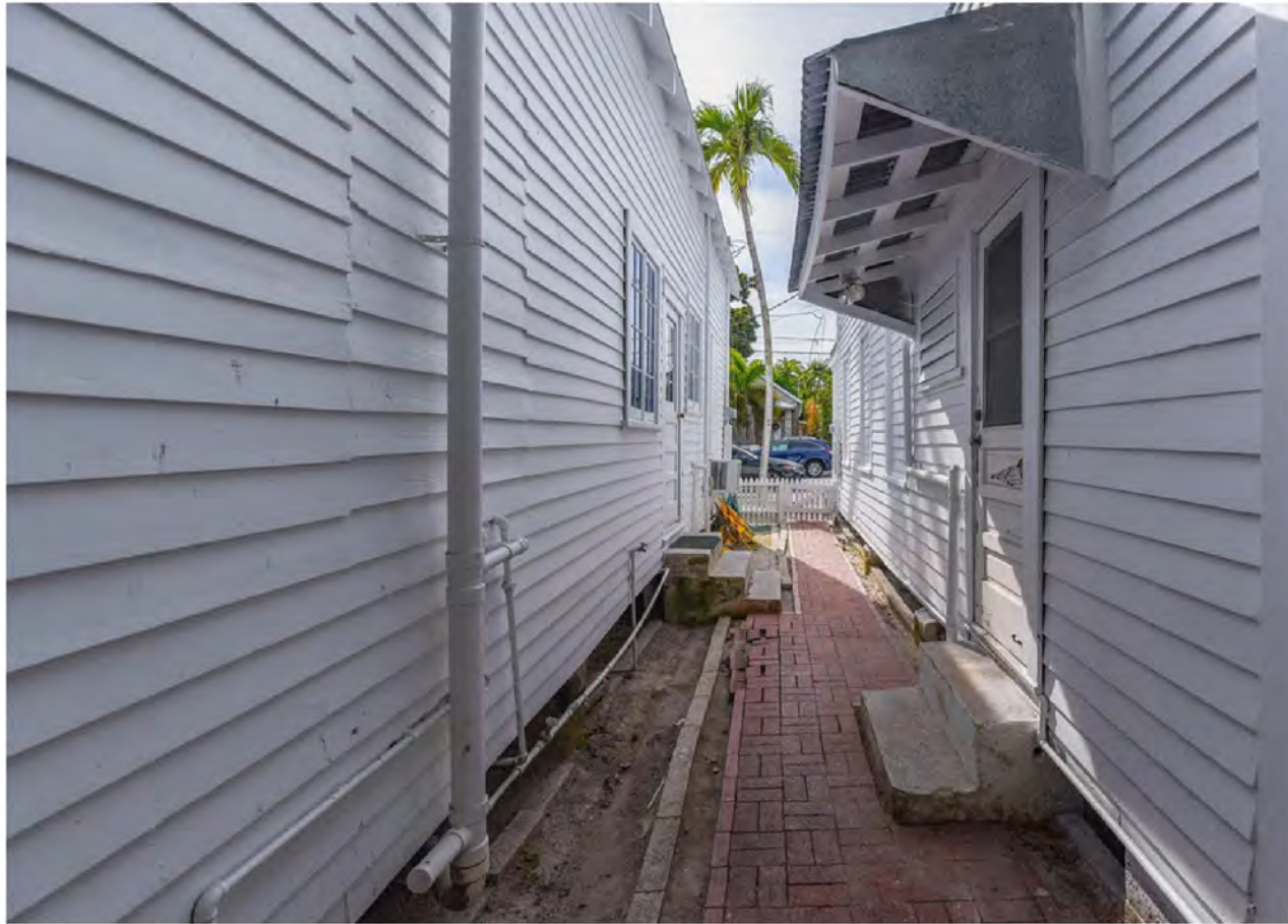
PREVIOUS NORTH SIDE FACADE, FACING STREET
