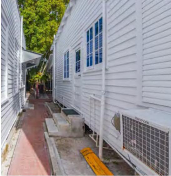
North facade prior to alteration.
