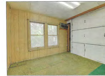
19 BACK ROOM A0.1 PREVIOUS INTERIOR
