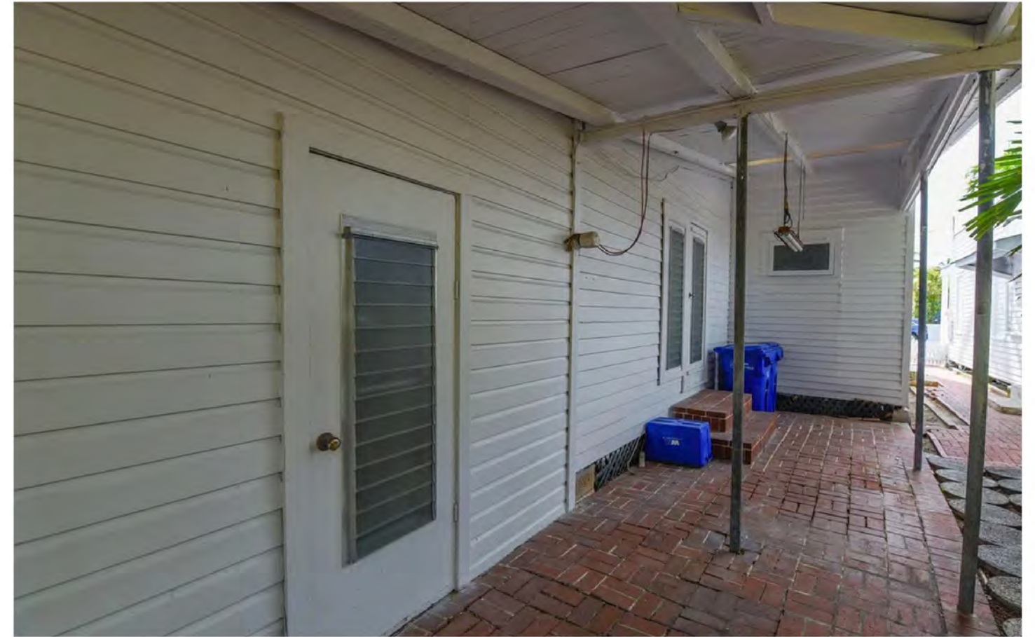
PREVIOUS REAR FACADE, AT NON-HISTORIC ADDITION
