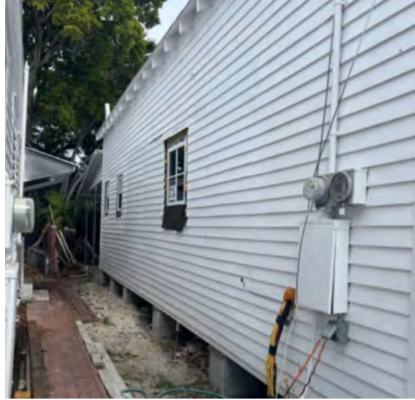
North facade after alteration.
