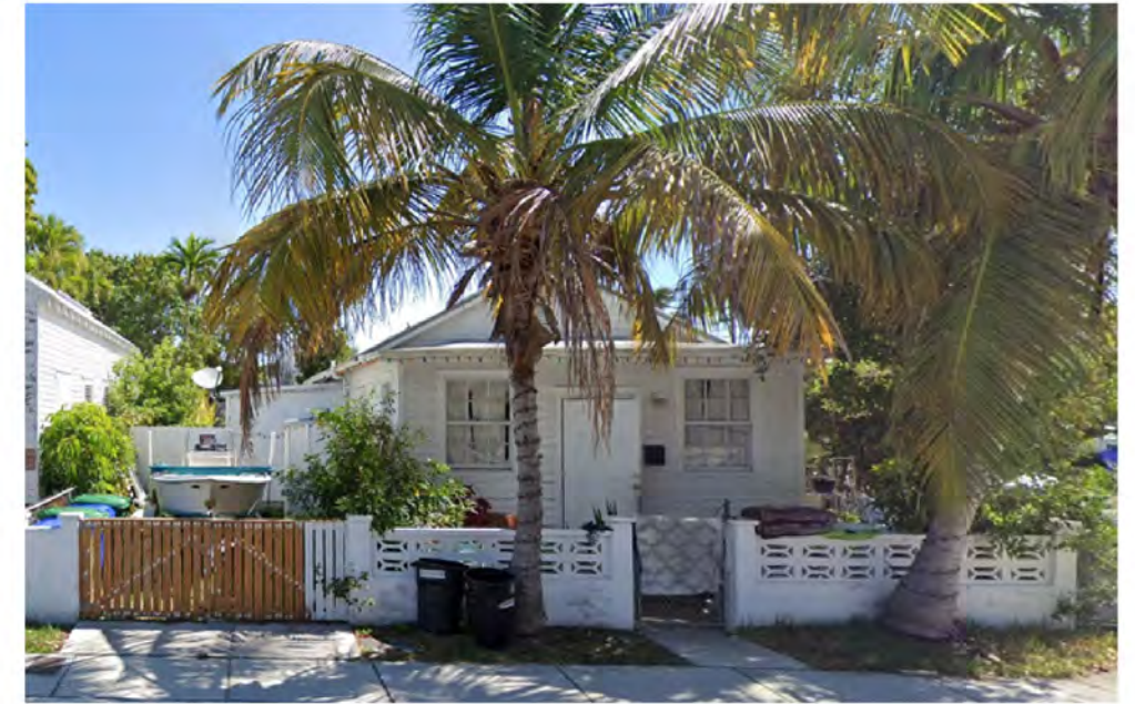
1025 GRINNELL EXAMPLE OF 2 OVER 2 WINDOWS ON PRIMARY FACADE
