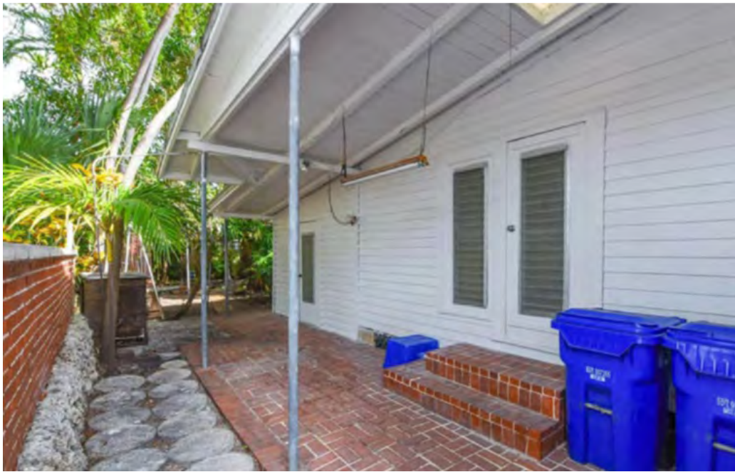
Addition prior to alteration
