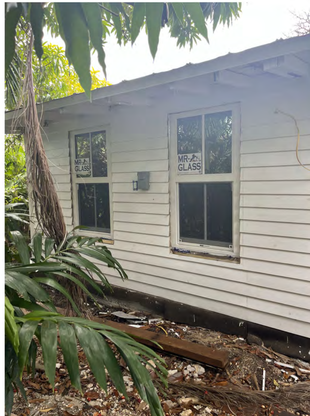
CURRENT REAR OF HOUSE, NEW ADDITION
