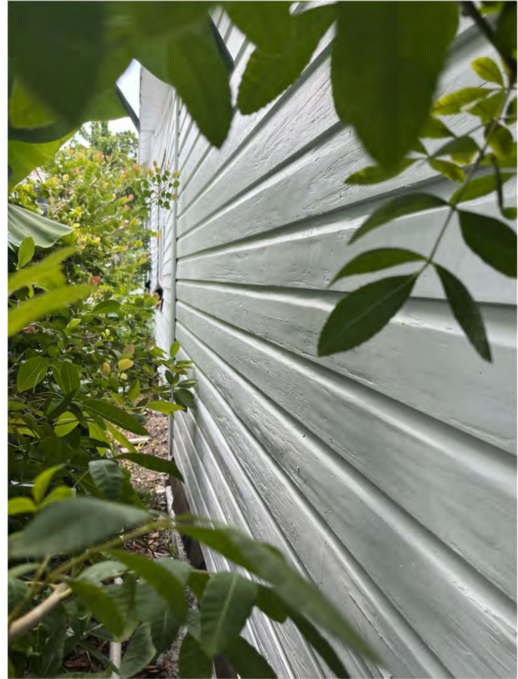
CURRENT SOUTH SIDE FACADE, FACING STREET (OBSTRUCTED BY NEIGHBORING HOUSE)
