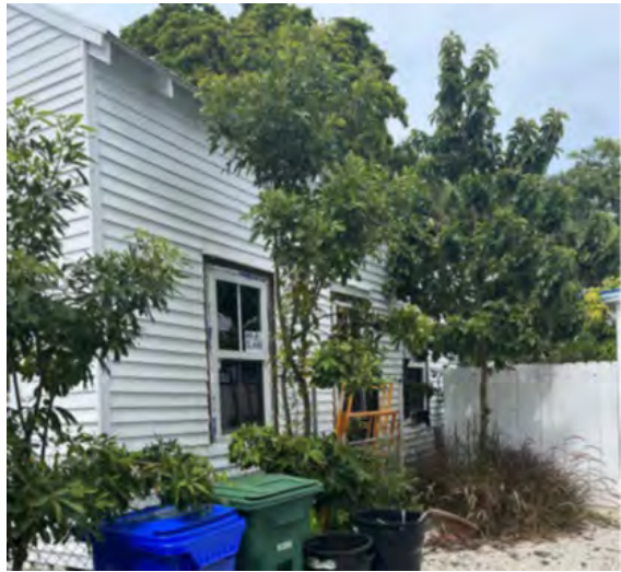
South facade with alteration.
