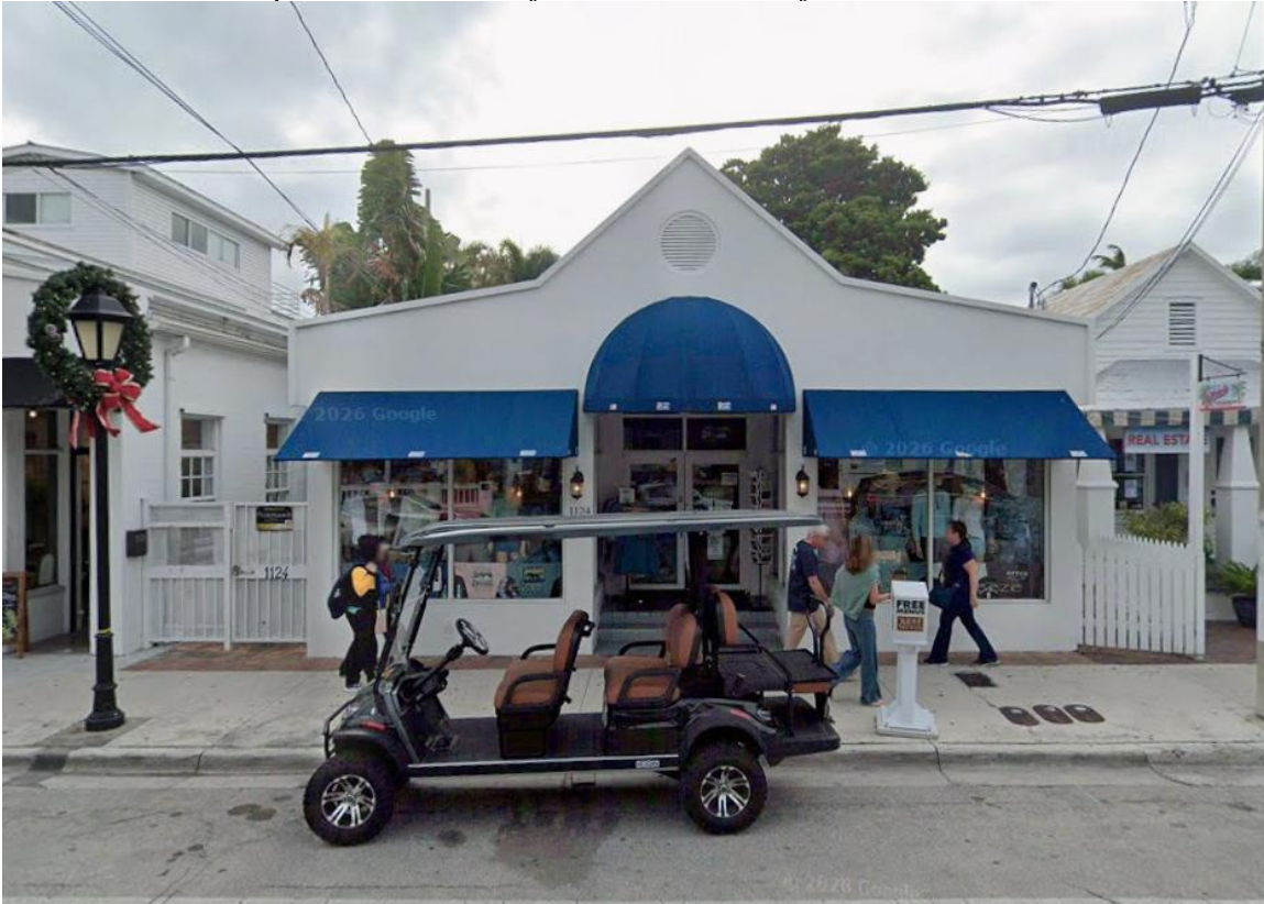
1124 Duval Street: permitted in 2004 for entrance, 2005 for windows
